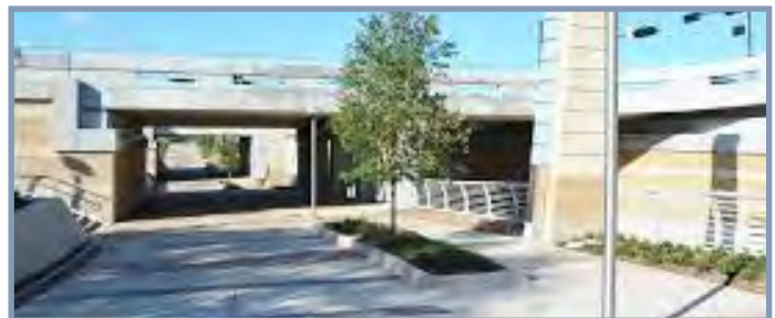
Tunnel connecting Texas A&M campus under an active railroad and street. Klotz Associates.
