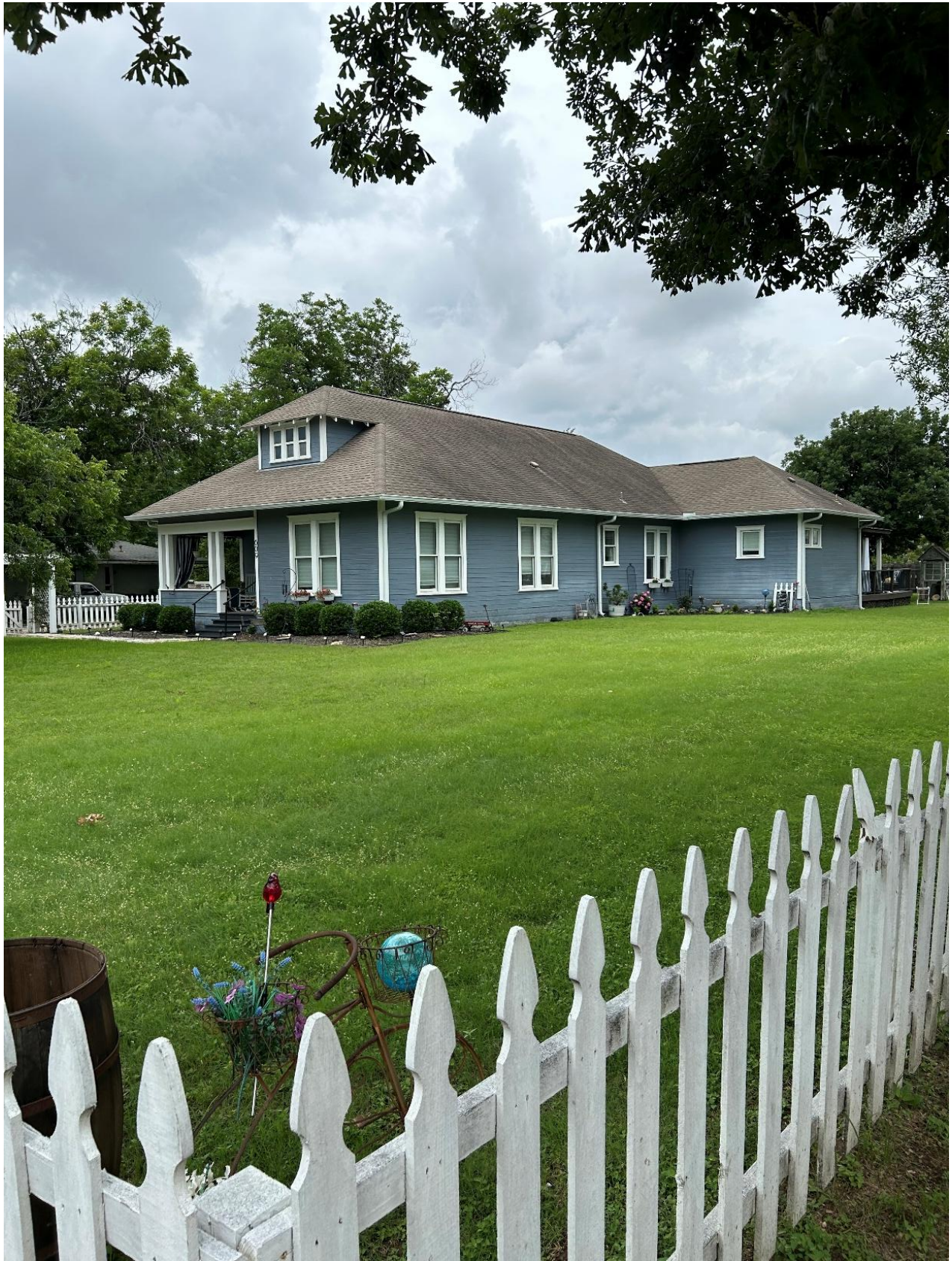
609 North FM 1660 Facing South West
