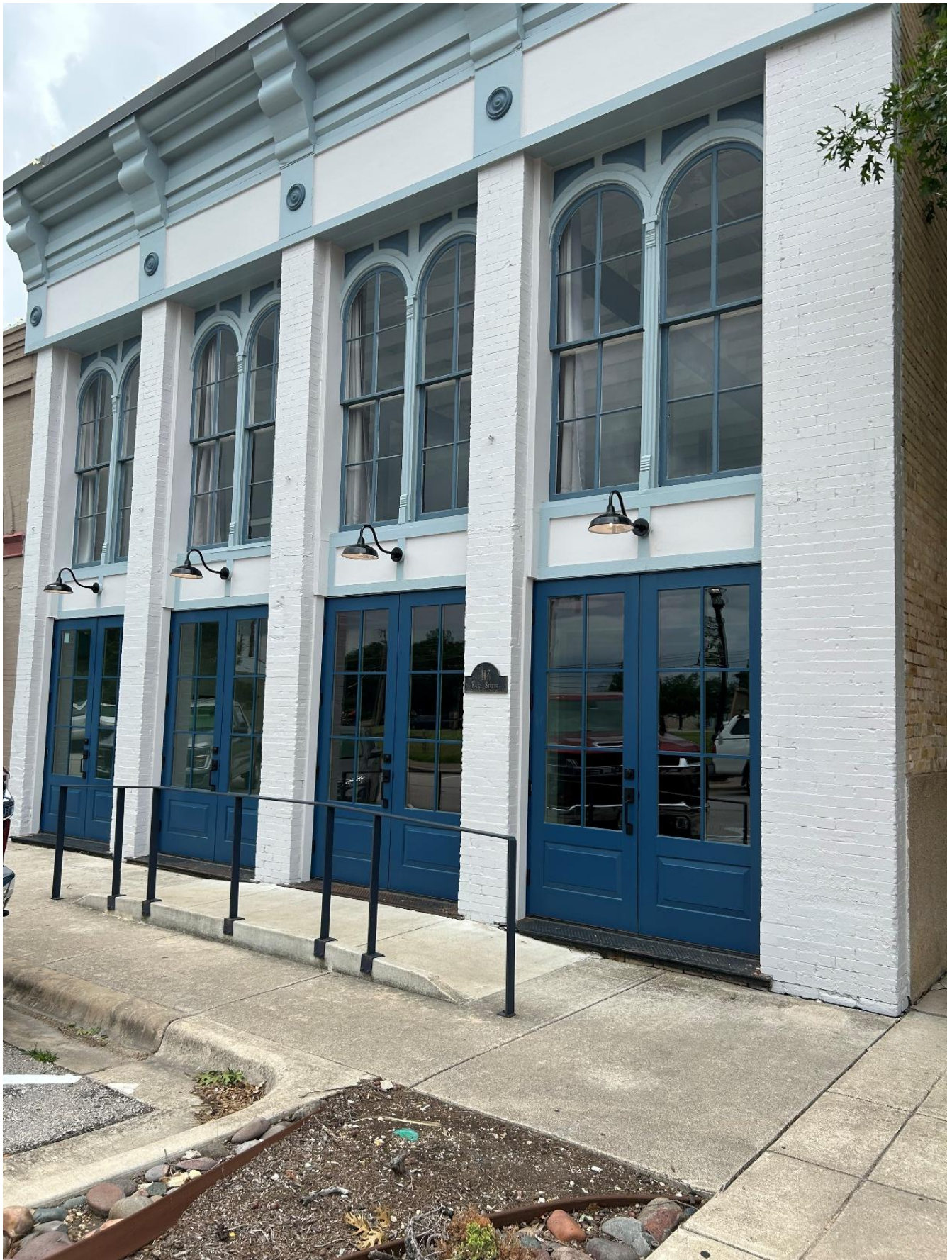
117 East Street Facing West
