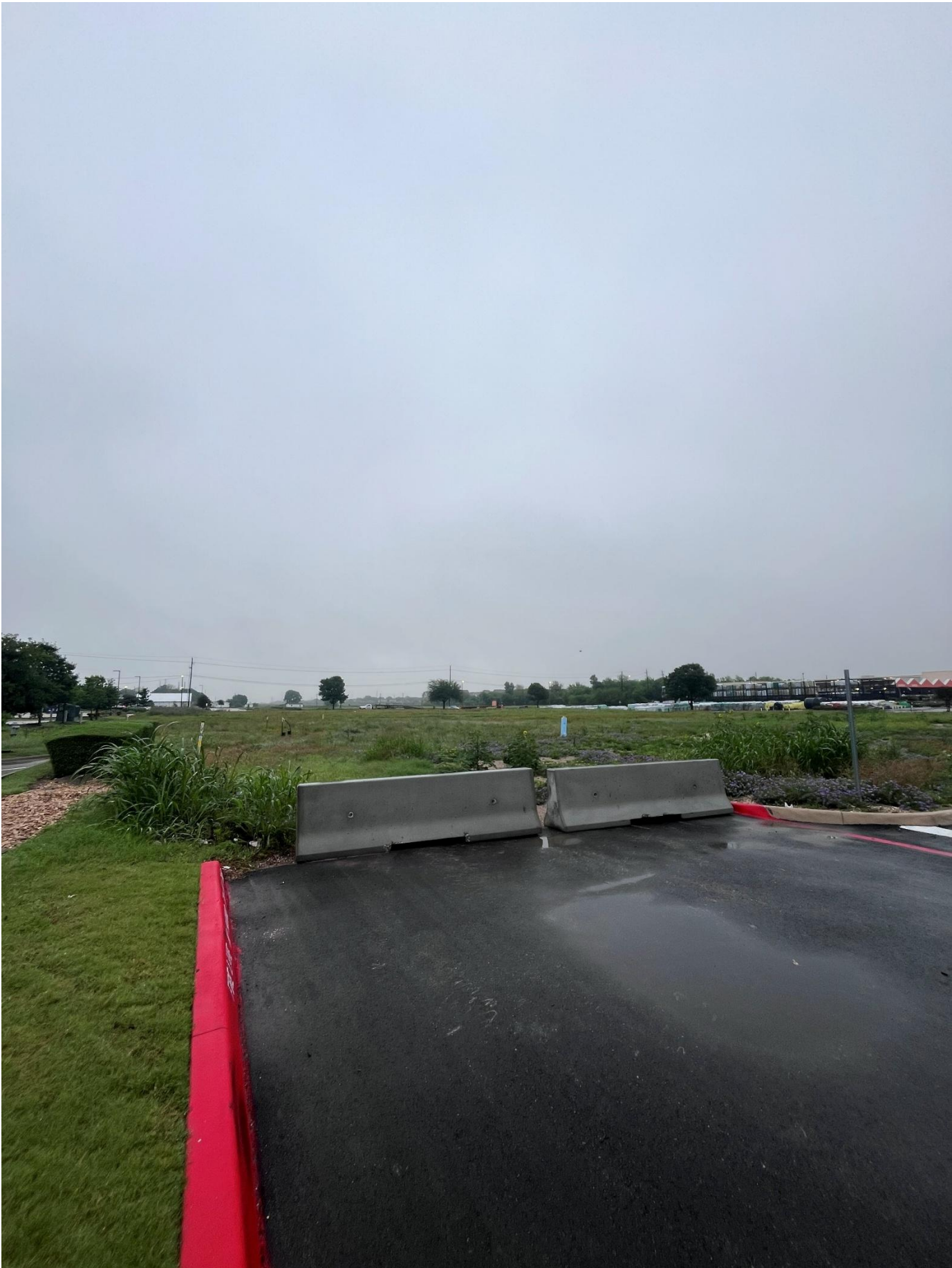
Southern Curb Cut Accessed Via Panera
