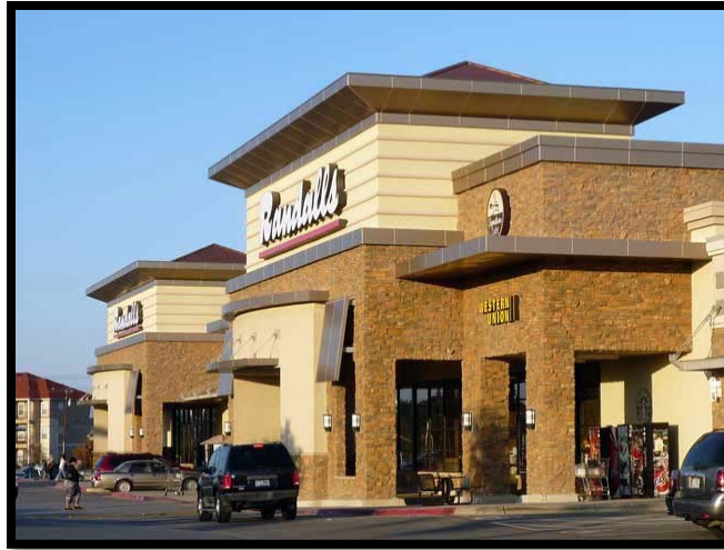
Figure 305.7-5: Primary Building Entrance
