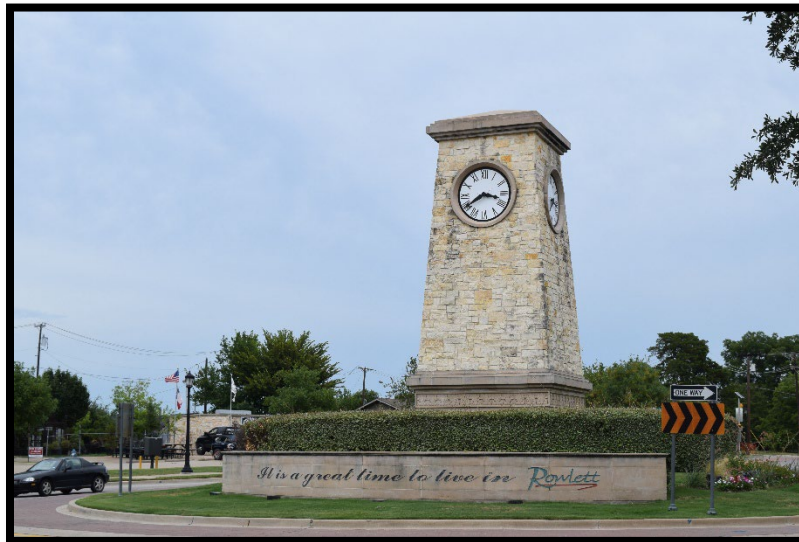
Figure 303.8-5 Clock Tower Example
