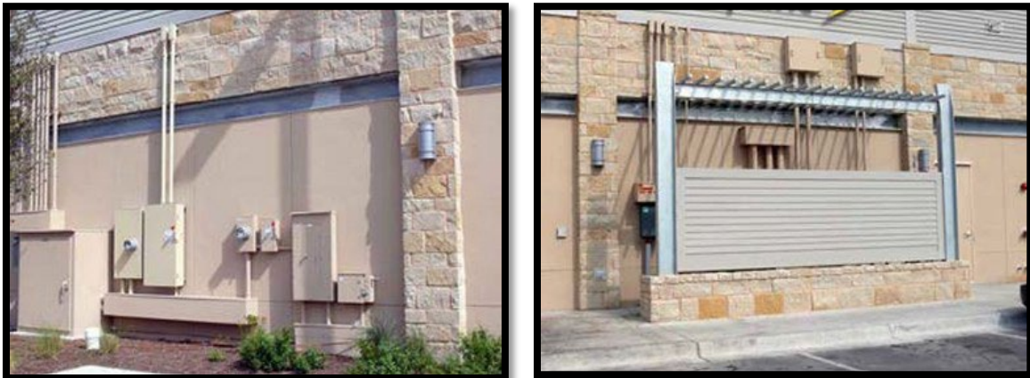
Figure 305.7-14: Utility Equipment Screening Standards
