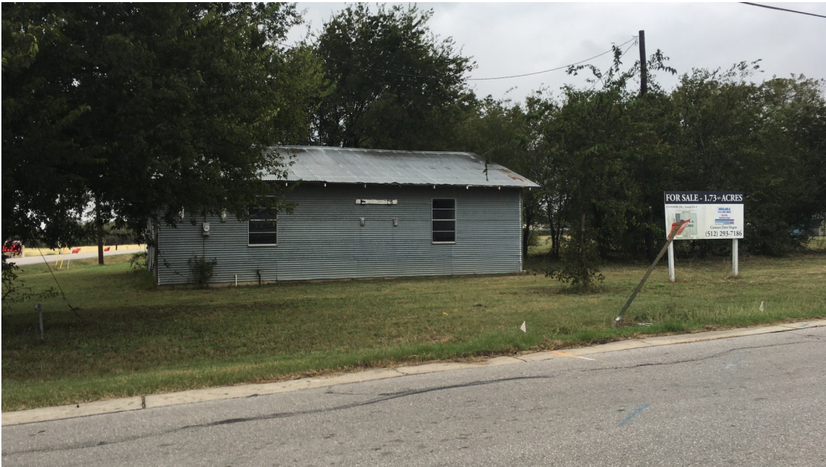
View of the subject property from E. Front Street, facing south
