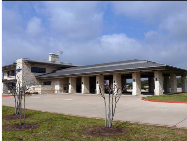
Drive-through architecturally integrated into host structure
