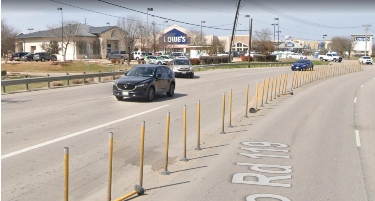
Figure 2. Traffic delineators on Ed Schmidt Blvd (source: Google Street View)
