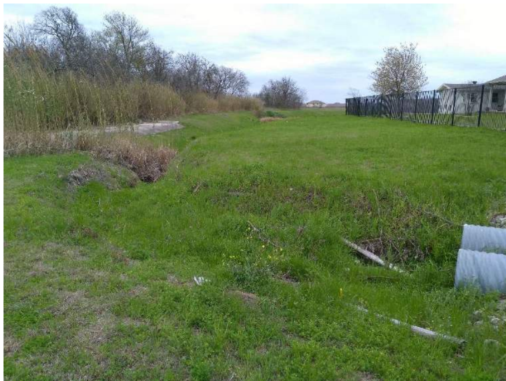
SOUTH DETENTION POND
