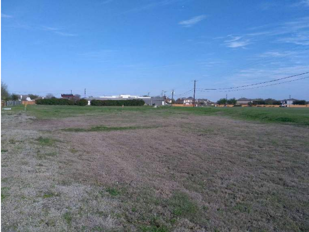
OVERALL VIEW OF DETENTION POND (LOOKING EAST)
