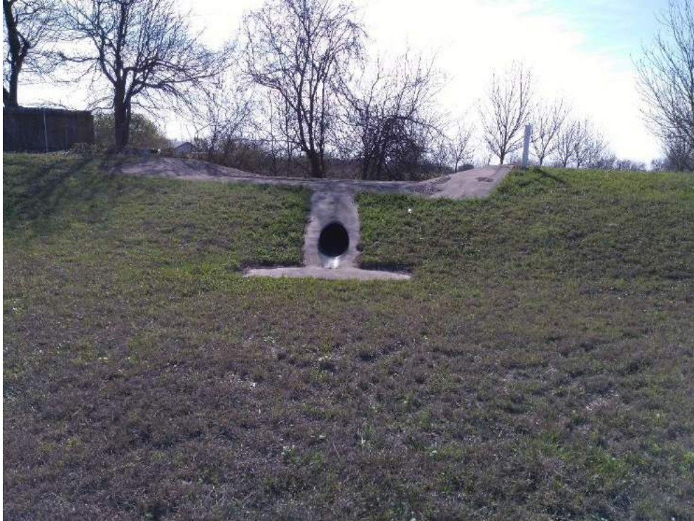
OVERFLOW STRUCTURE (LOOKING FROM UPSTREAM)
