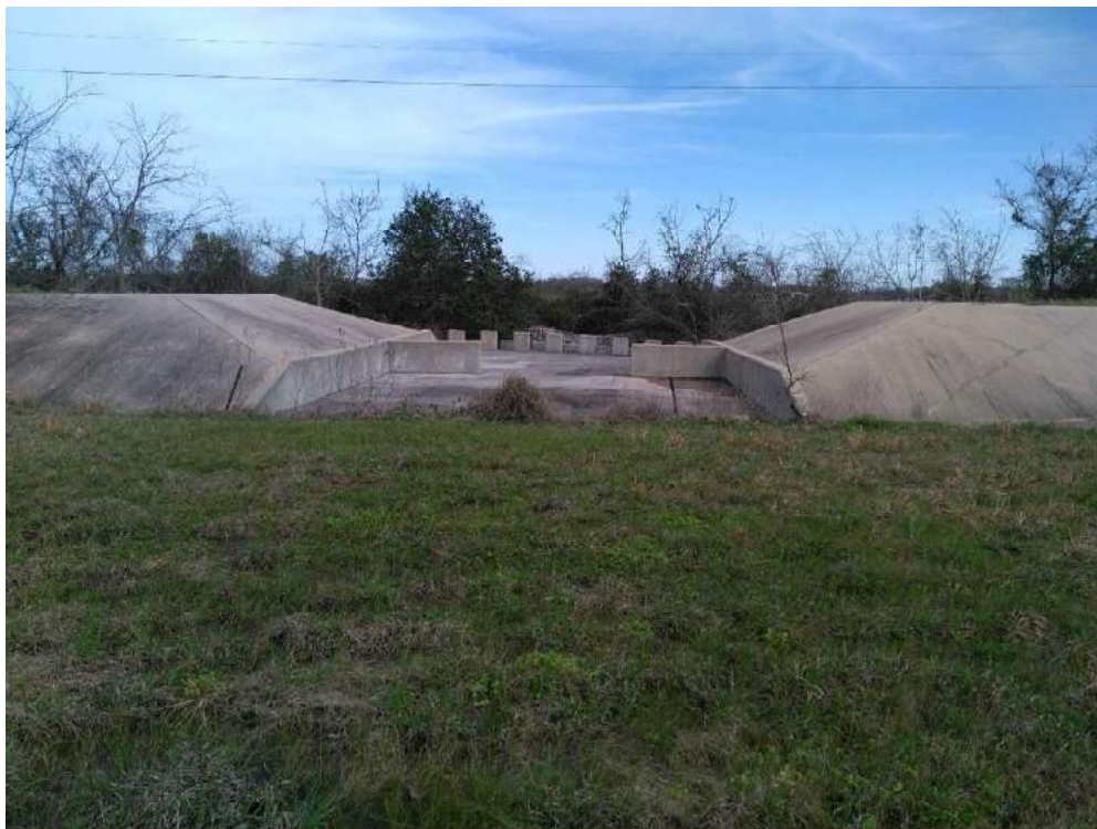
OVERFLOW STRUCTURE (LOOKING EAST)
