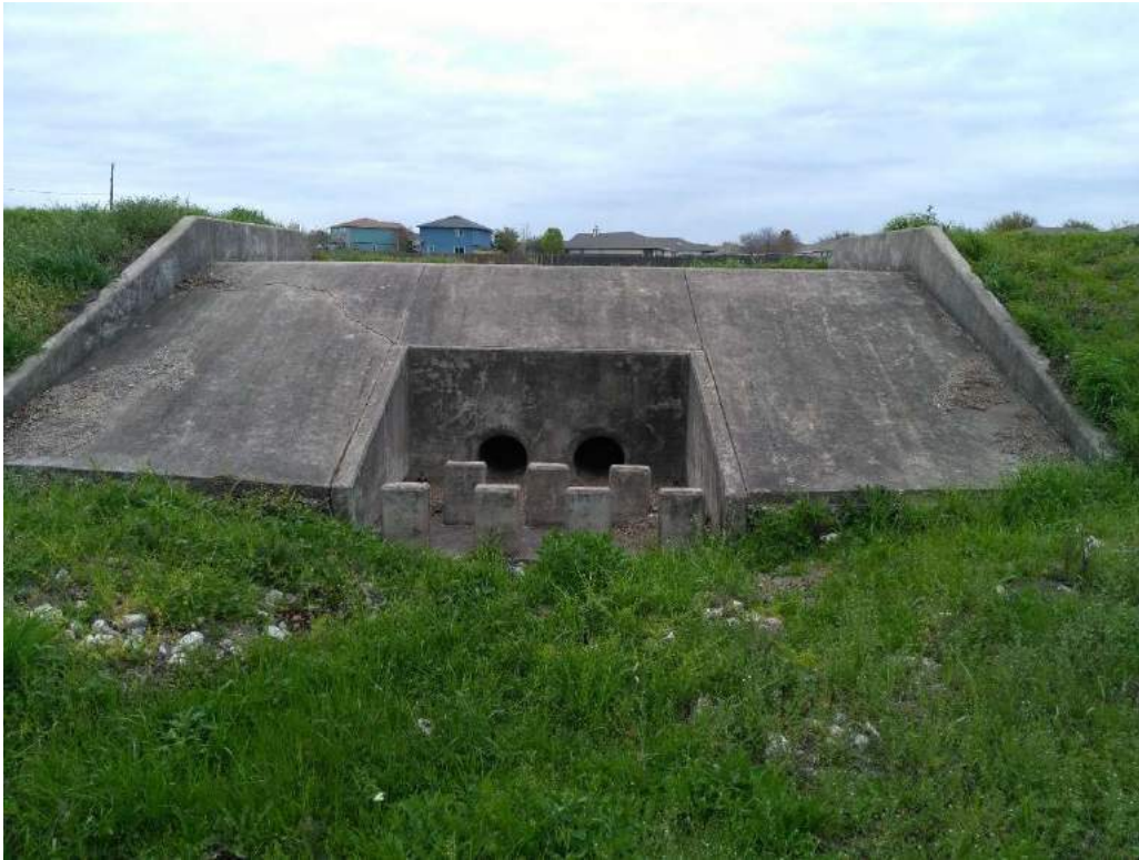
OVERFLOW STRUCTURES (LOOKING FROM DOWNSTREAM)
