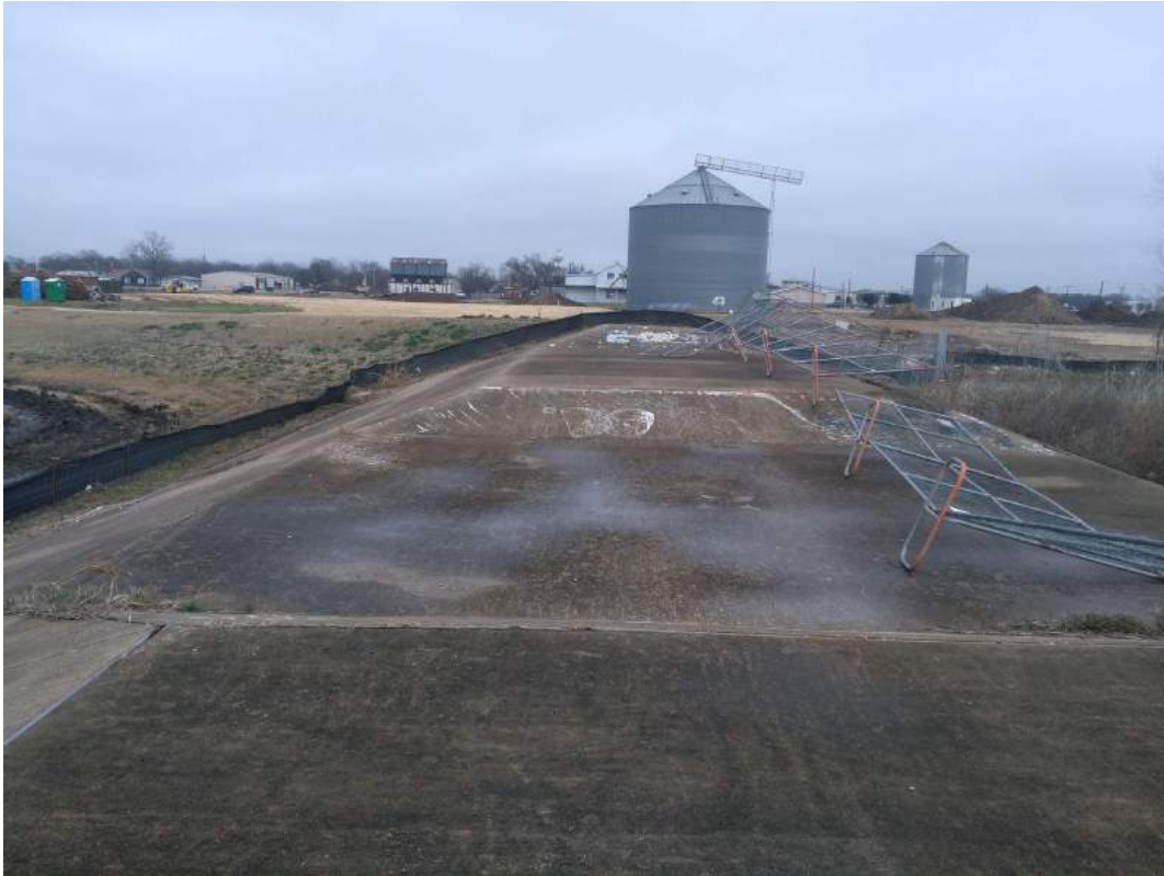
OVERFLOW STRUCTURE (LOOKING EAST)
