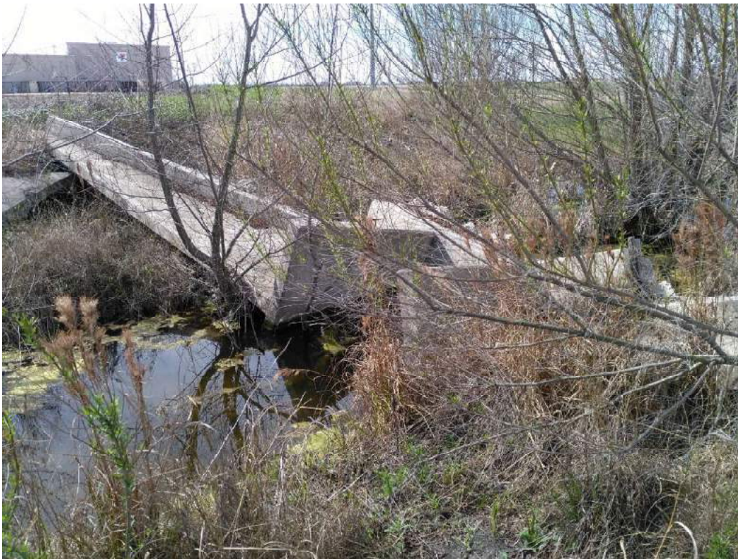
TIPPED OUTFALL STRUCTURE
