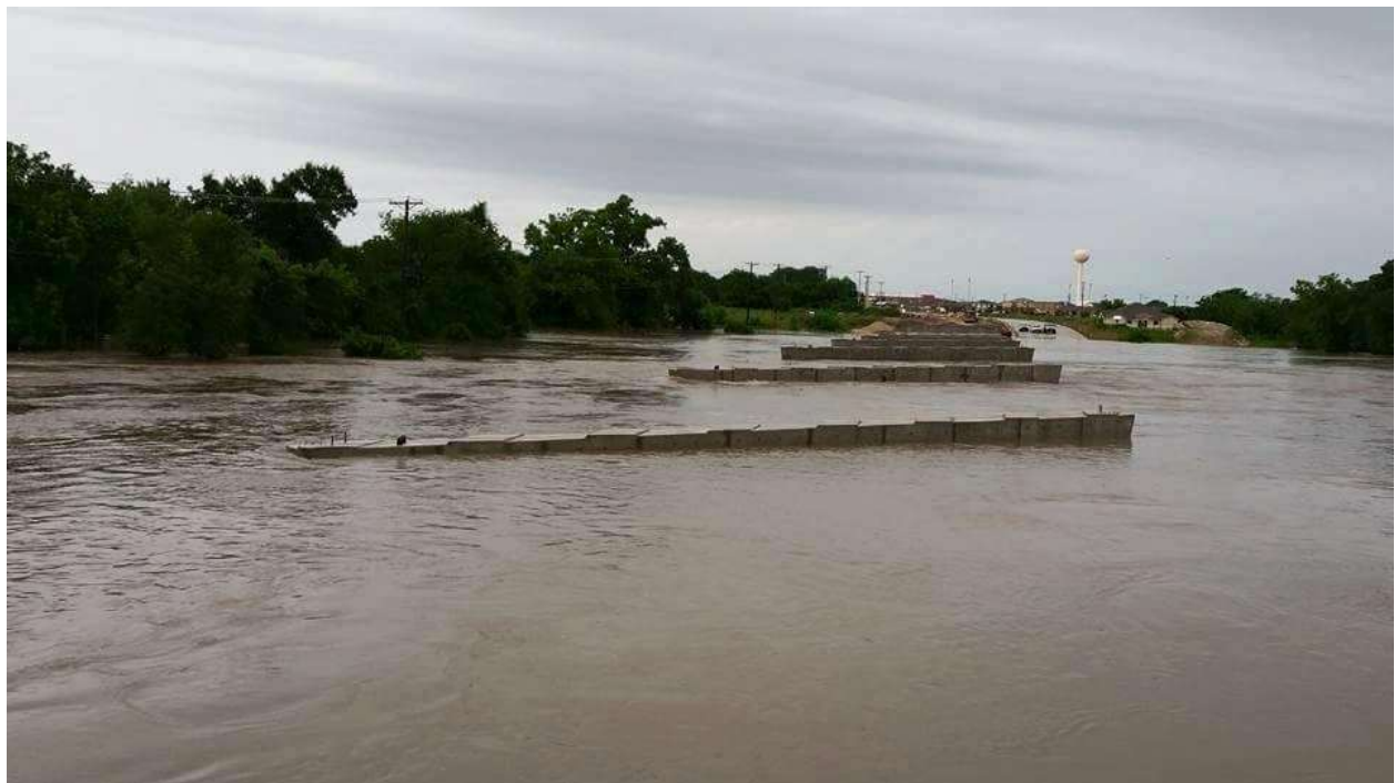
Figure 1 Brushy Creek and FM 685/Chris Kelley Boulevard bridge support structure under construction during May 2015 Memorial Day flood event. Top of bent caps can be seen just above Brushy Creek flood water. Bridge has subsequently built and in operation.
