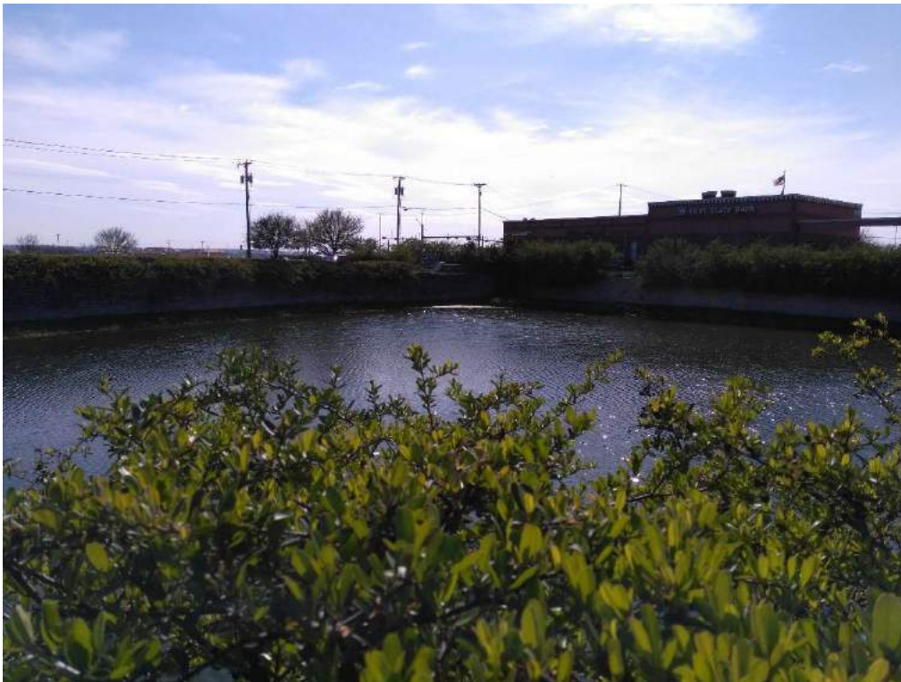
OVERALL VIEW OF DETENTION POND (LOOKING SOUTHWEST)
