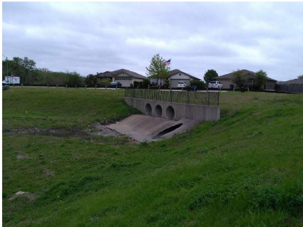
DETENTION POND (LOOKING EAST)
