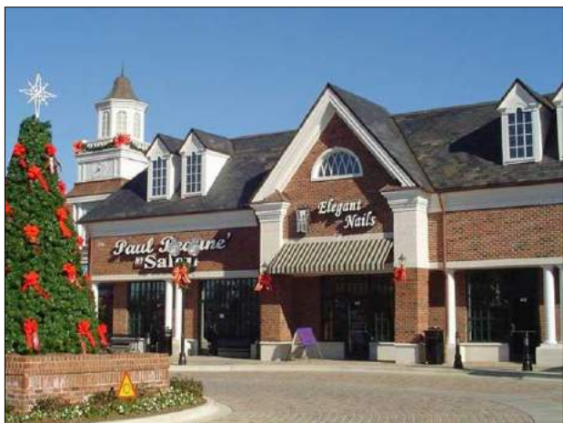
Peaked roof form, canopy, display windows, projections
