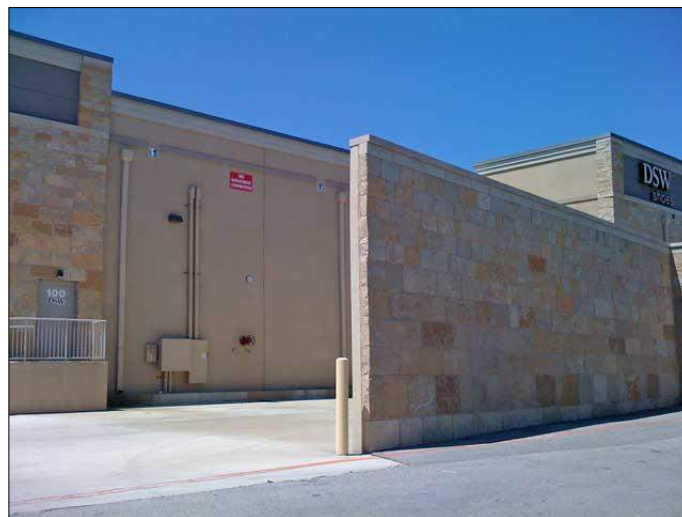
Effective use of wing wall used to screen loading dock
