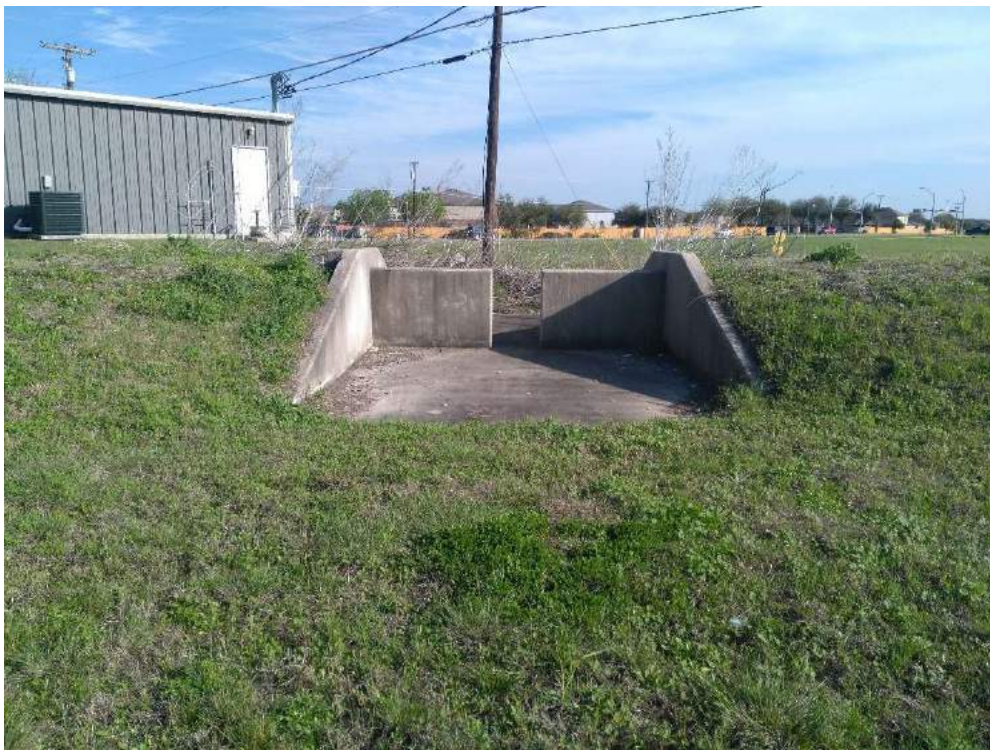
OVERFLOW STRUCTURES (LOOKING FROM UPSTREAM)
