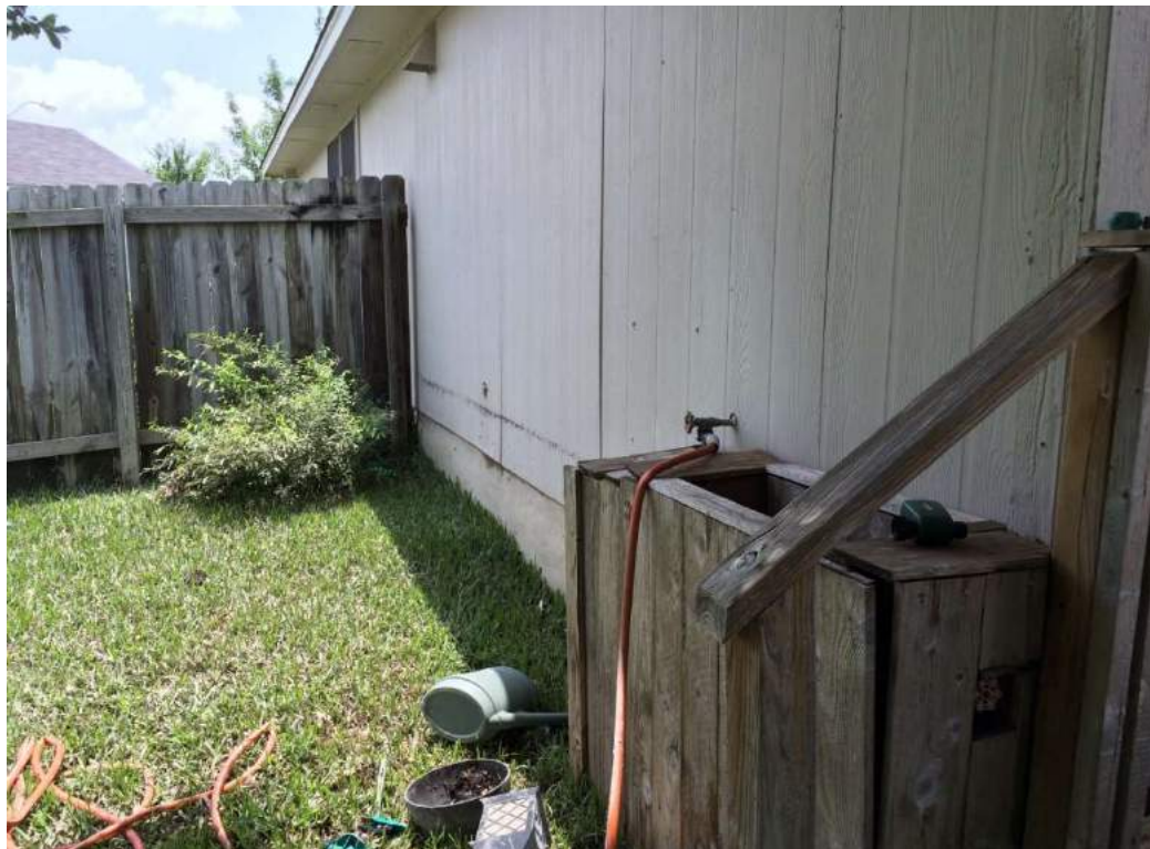
Figure 3 Flood elevation appears on residential structure Located at 522 Meadowside Drive in the Creekbend Subdivision after May 2015 Memorial Day flood event
