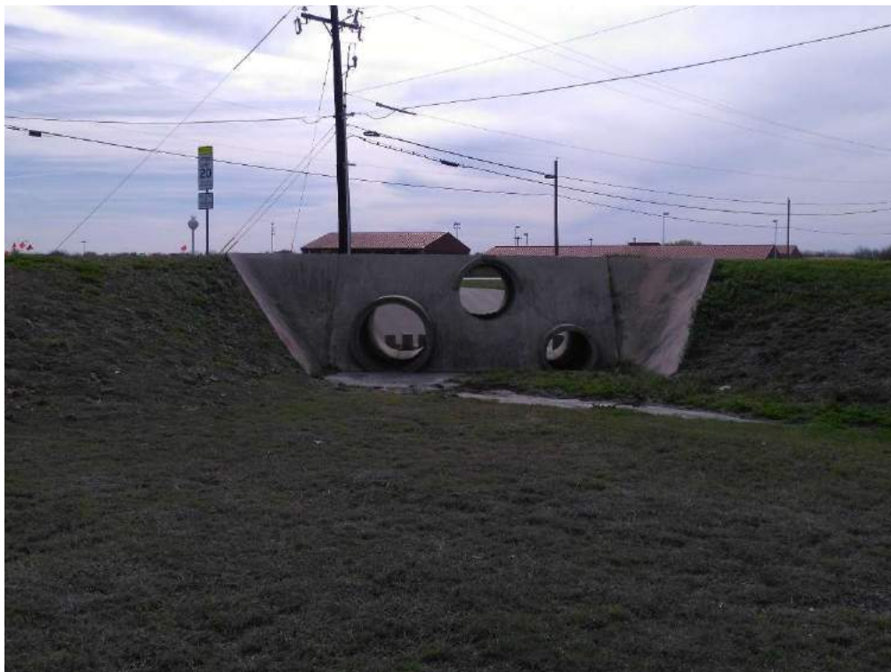
OVERFLOW STRUCTURE (UPSTREAM SIDE)
