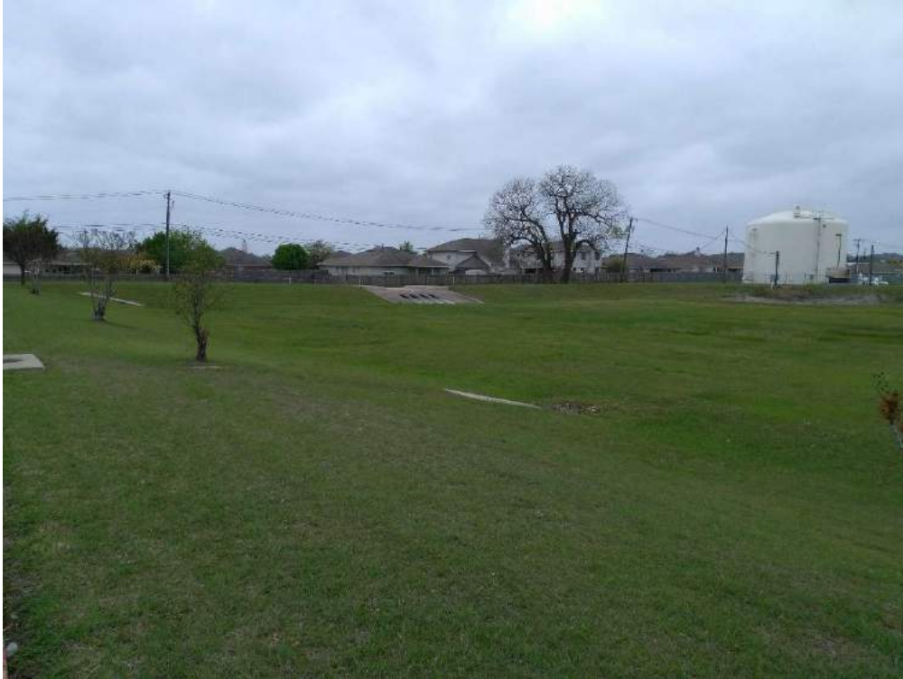
OVERALL VIEW OF ELEMENTARY SCHOOL DETENTION POND (LOOKING WEST)
