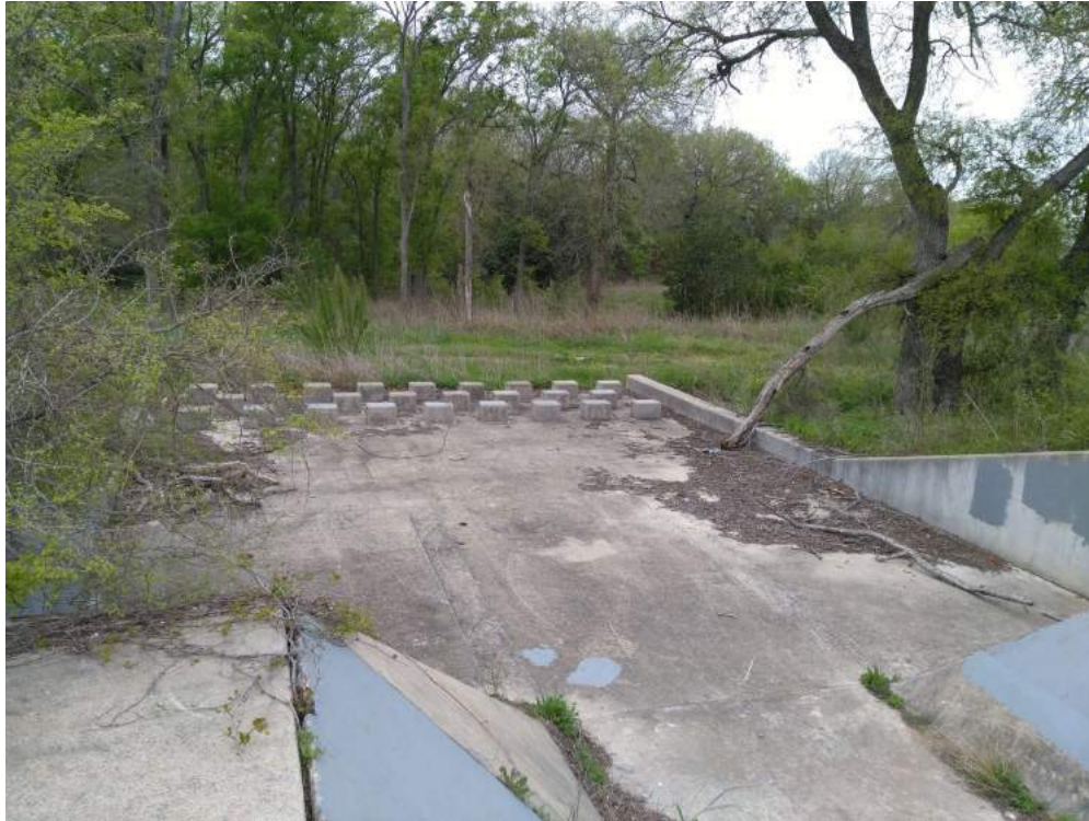
LOOKING DOWNSTREAM AT OVERFLOW STRUCTURE
