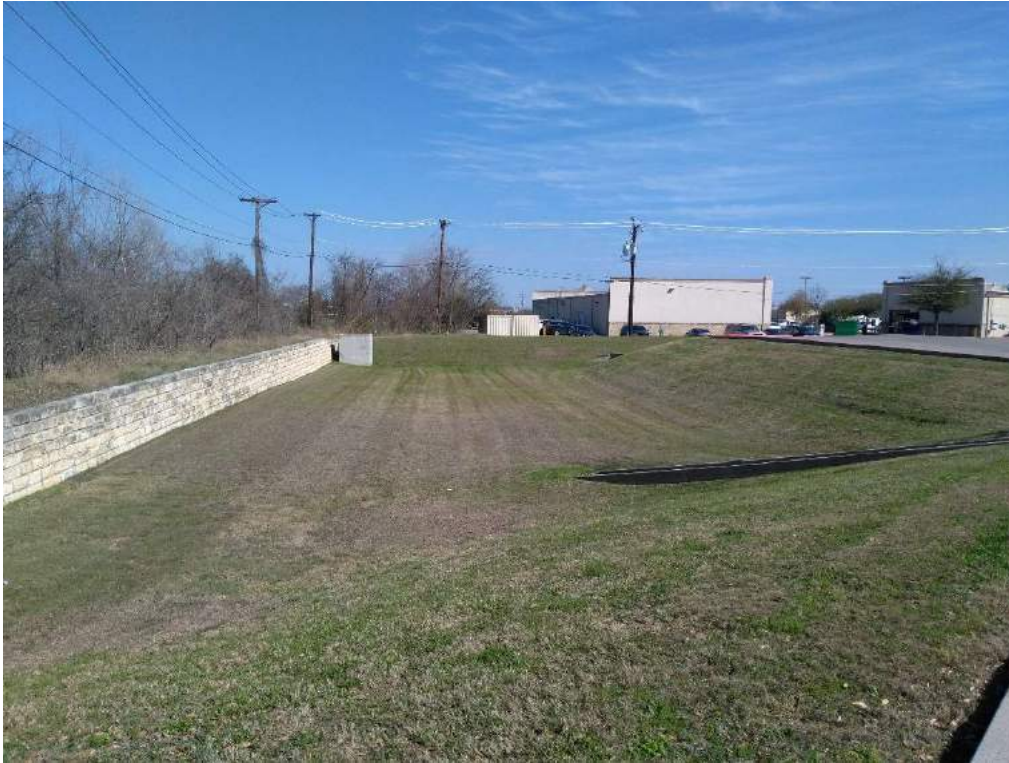
OVERALL VIEW OF DETENTION POND (LOOKING EAST)
