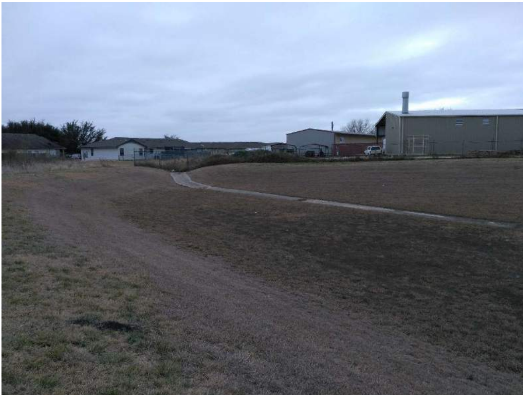
OVERALL VIEW OF DETENTION POND (LOOKING SOUTH)
