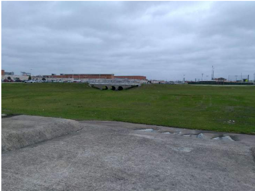
OVERALL VIEW OF DETENTION POND (LOOKING NORTH)
