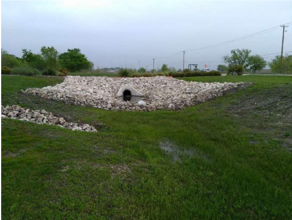
DETENTION POND (LOOKING NORTH)
