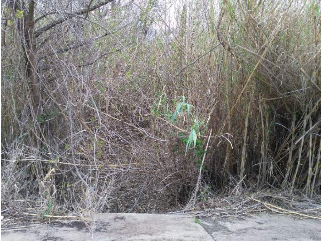
OVERFLOW WEIR (LOOKING AT DOWNSTREAM)
