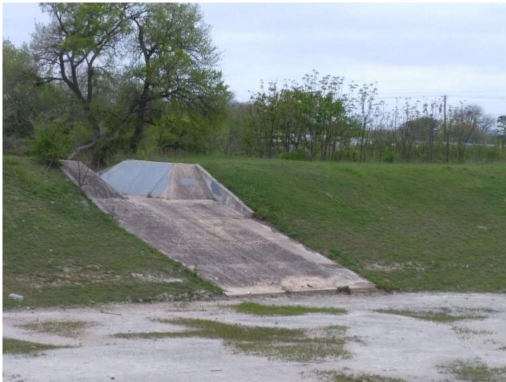
LOOKING AT OVERFLOW STRUCTURE
