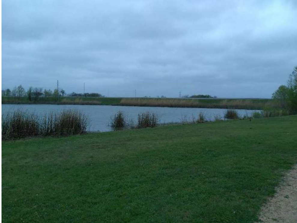
OVERALL VIEW OF WCID #20 DAM (LOOKING NORTH)
