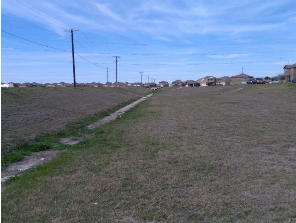
OVERALL VIEW OF DETENTION POND (LOOKING NORTH)
