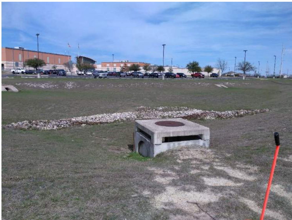
OVERFLOW STRUCTURE (LOOKING NORTHEAST)
