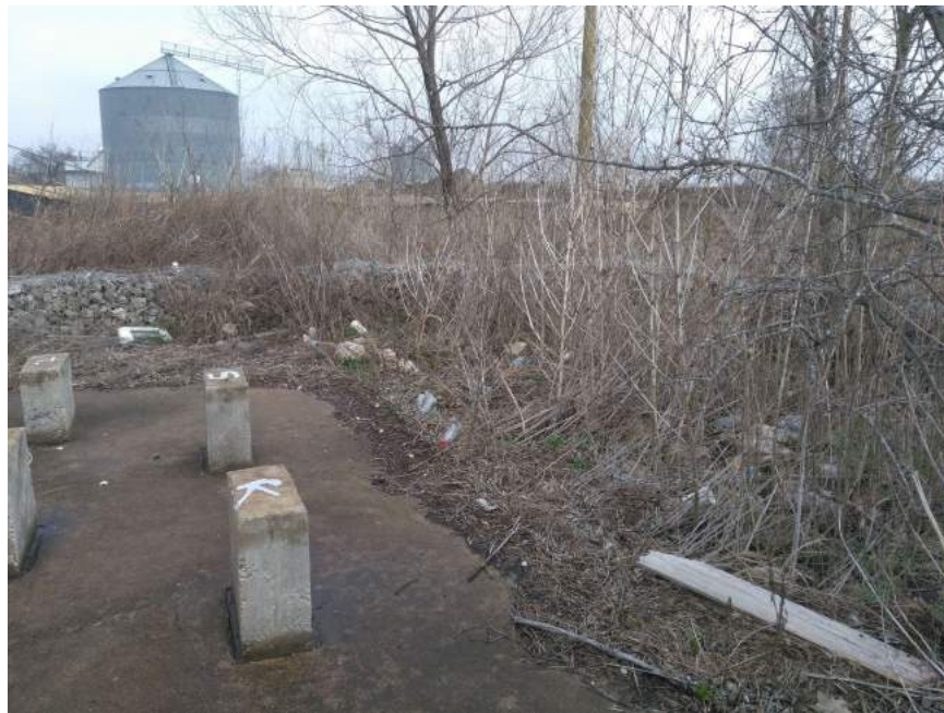
VEGETATION AND DEBRIS AT OUTFALL
