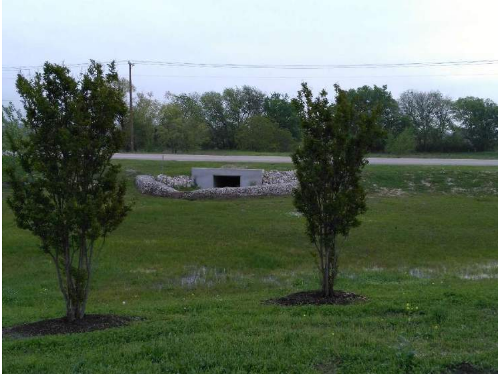
DETENTION POND (LOOKING EAST)
