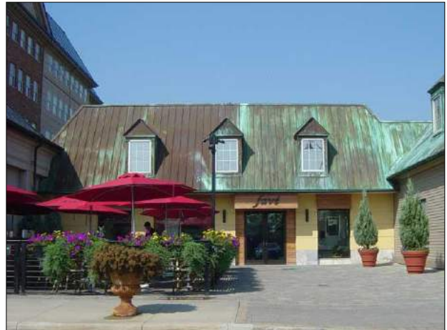
Outdoor patio, display windows
