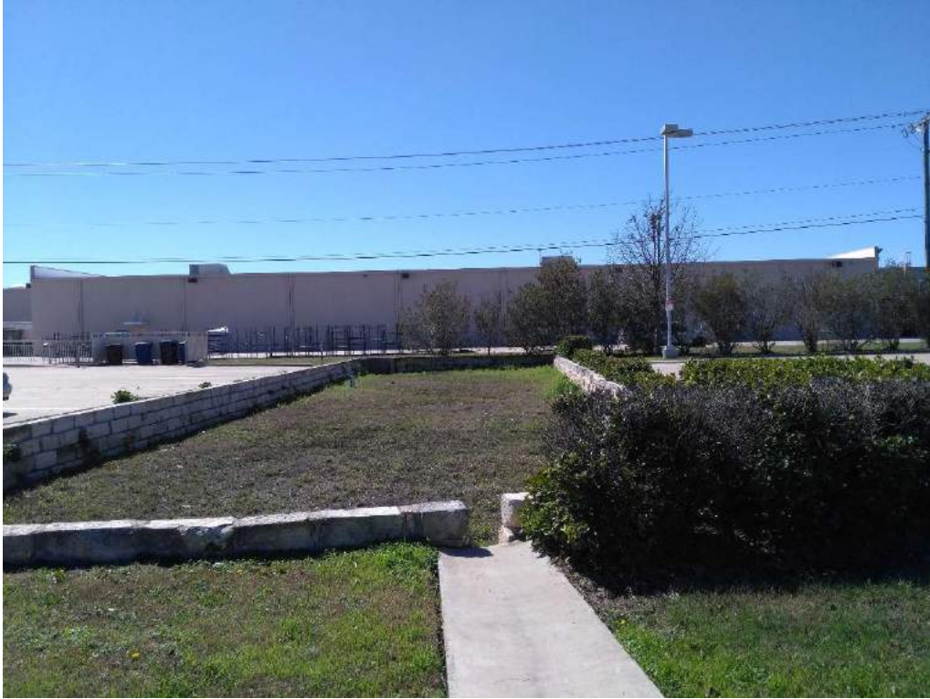
OVERALL VIEW OF DETENTION POND (LOOKING SOUTH)
