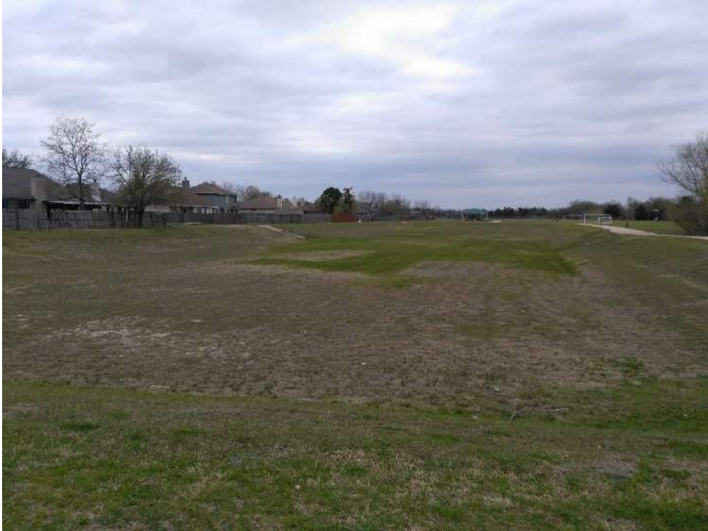
OVERALL VIEW OF DETENTION POND (LOOKING NORTH)
