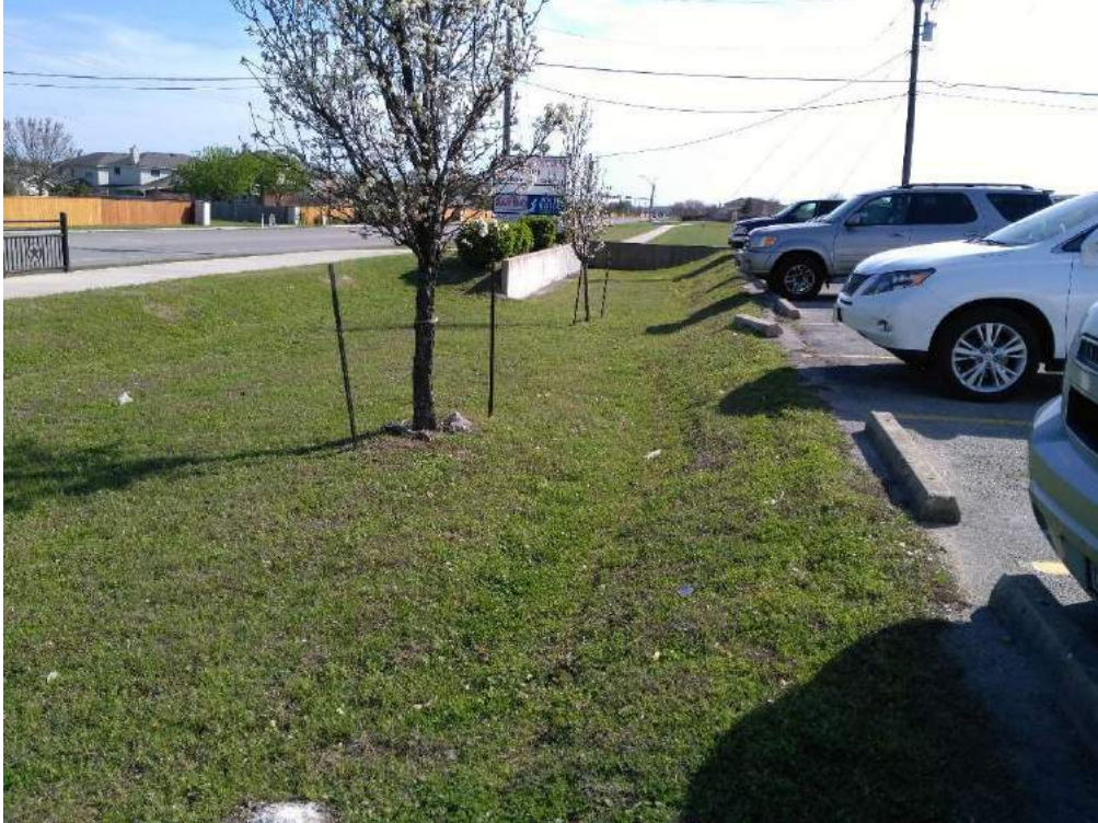
OVERALL VIEW OF DETENTION POND (LOOKING SOUTH)
