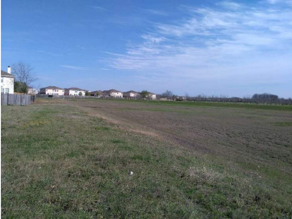
OVERALL VIEW OF DETENTION POND (LOOKING EAST)
