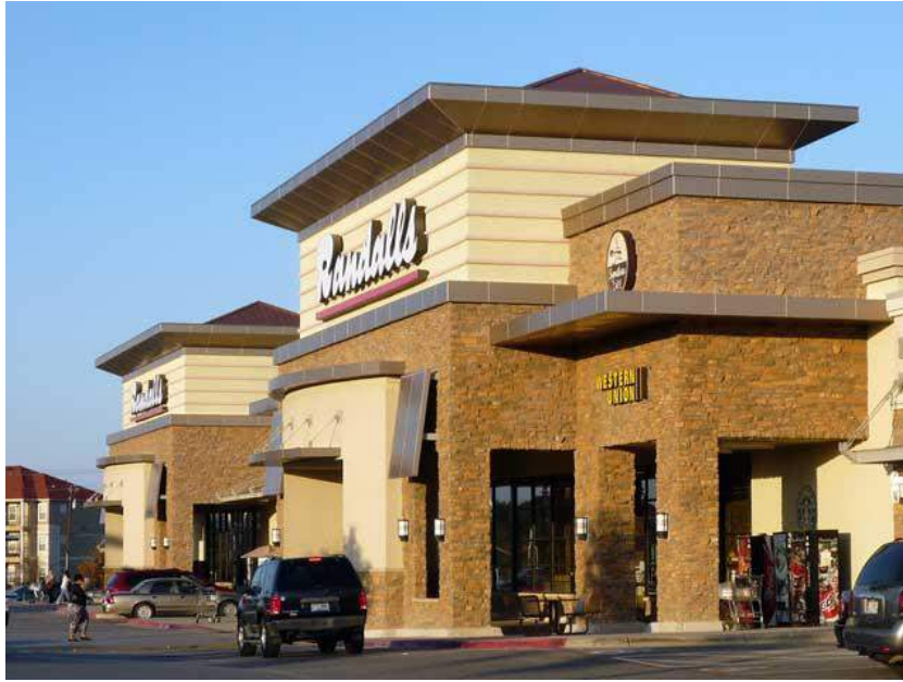
Well-defined building entrance
