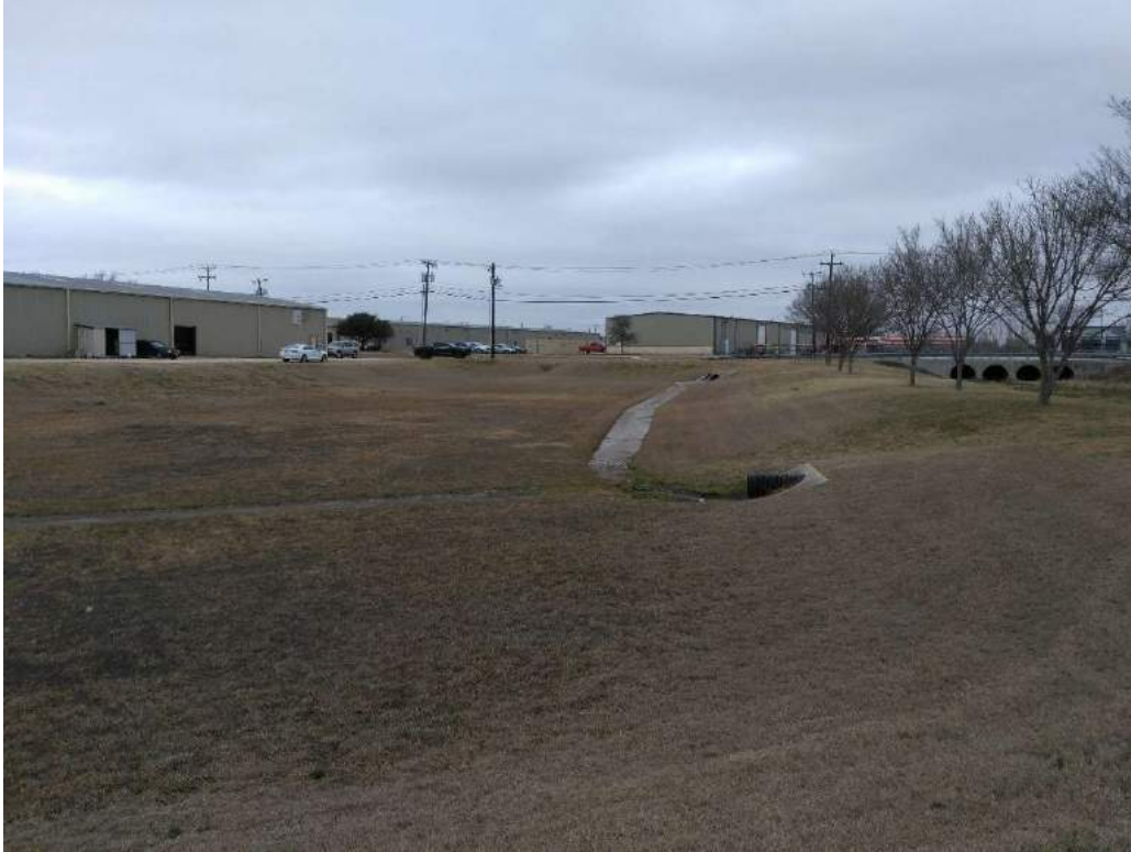
OVERALL VIEW OF DETENTION POND (LOOKING NORTH)
