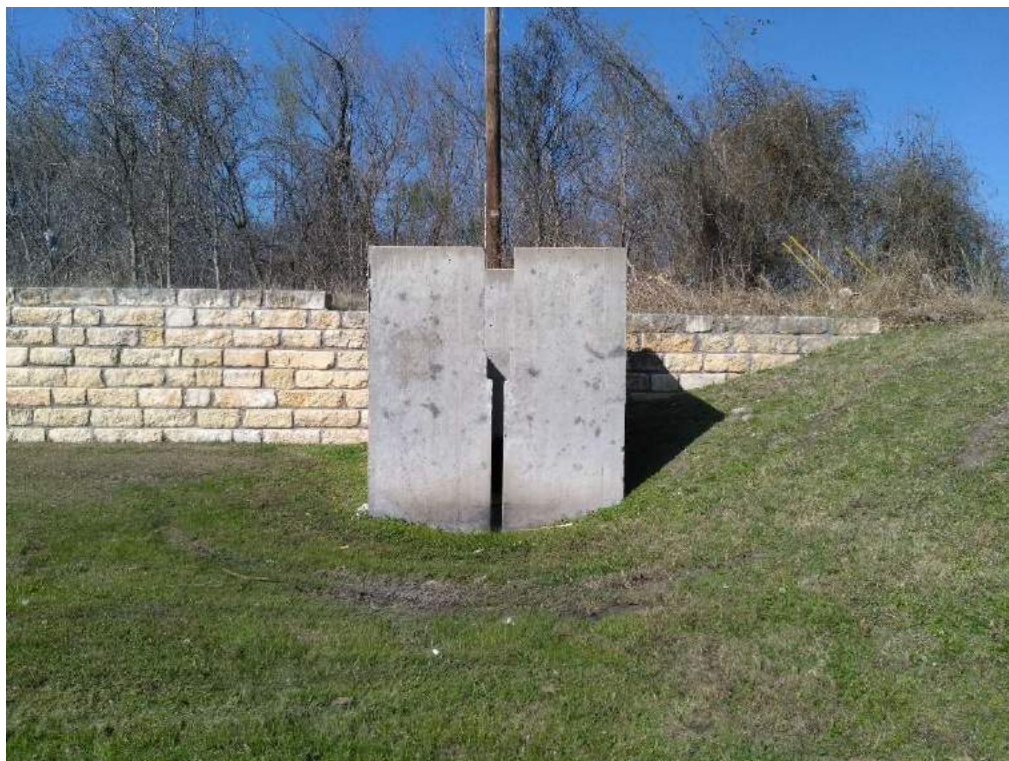
OVERFLOW STRUCTURES (LOOKING NORTH)
