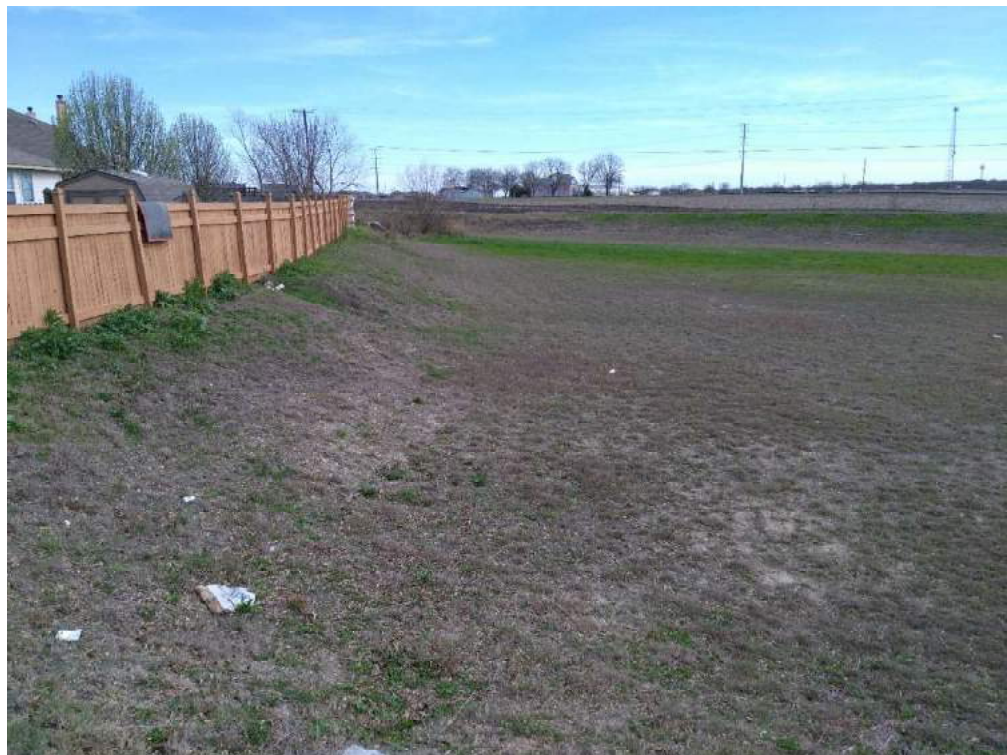
OVERALL VIEW OF DETENTION POND (LOOKING SOUTH)
