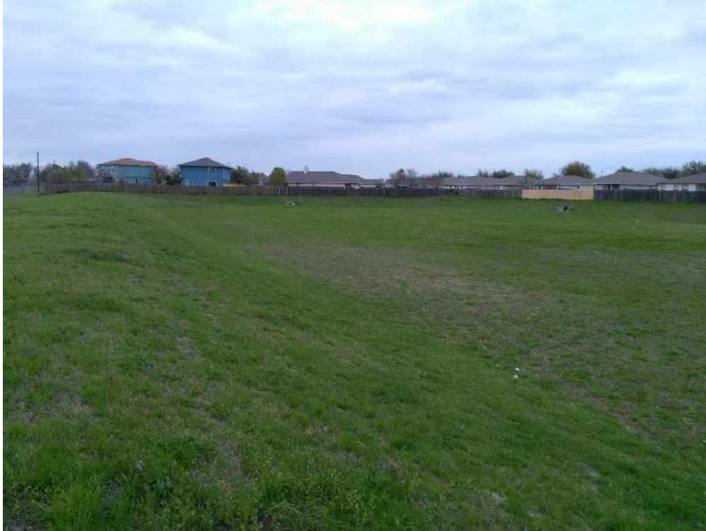
OVERALL VIEW OF DETENTION POND (LOOKING NORTH)
