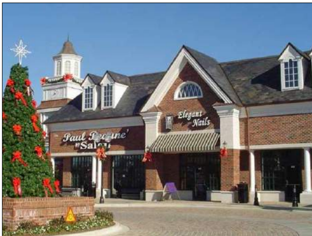
Peaked roof form, canopy, display windows, projections
