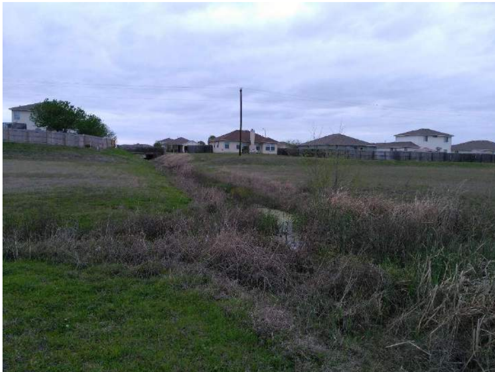
TRICKLE CHANNEL, OVERGROWN VEGETATION AND STANDING WATER
