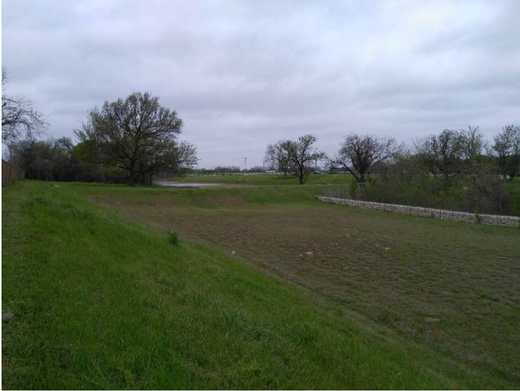
DETENTION POND (LOOKING WEST)
