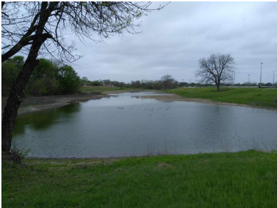
DETENTION POND (LOOKING WEST)
