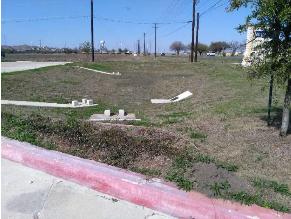
OVERALL VIEW OF DETENTION POND (LOOKING NORTH)
