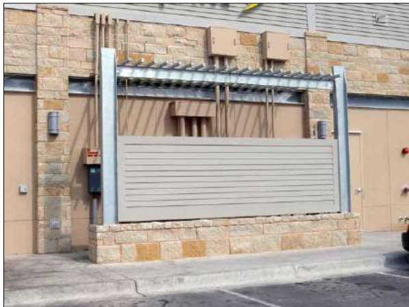
Utility equipment in more visible location screened by wing wall
