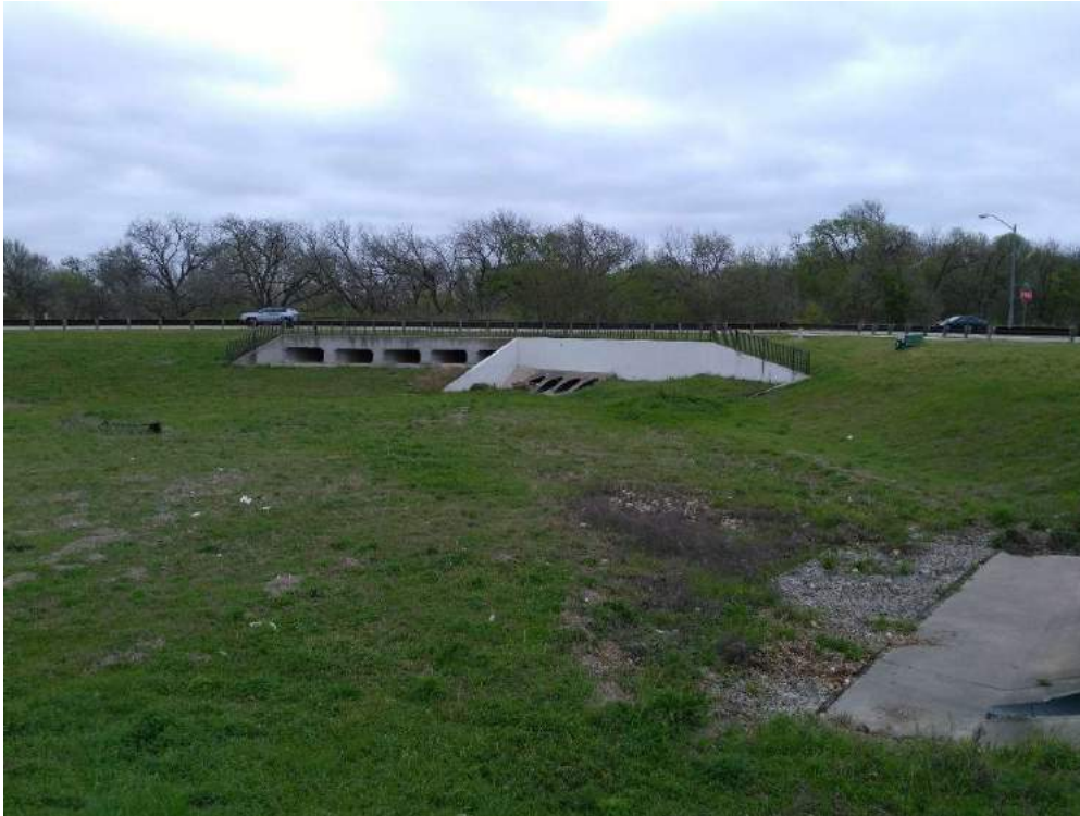
OVERALL VIEW OF DETENTION POND (LOOKING NORTH)
