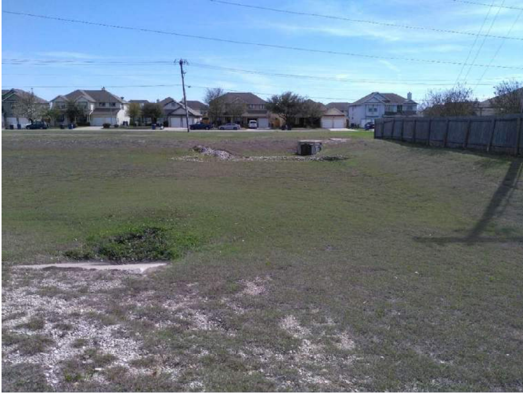
OVERALL VIEW OF DETENTION POND (LOOKING SOUTH)
