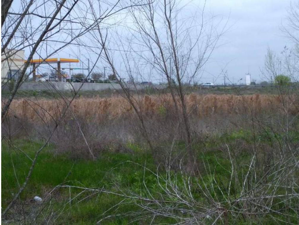
OVERALL VIEW OF DETENTION POND# 2 (LOOKING NORTH)
