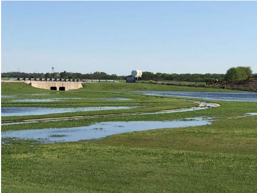
EAST DETENTION POND
