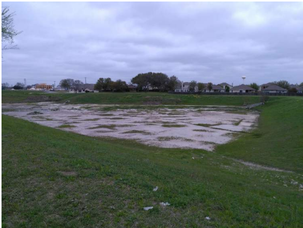
OVERALL VIEW OF DETENTION POND (LOOKING NORTHWEST)
