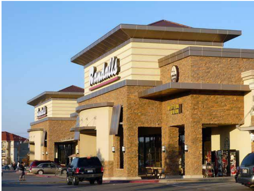
Well-defined building entrance
