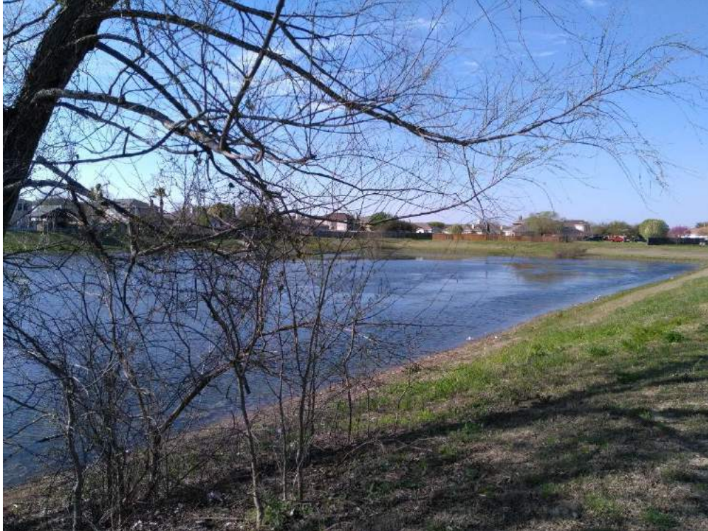
OVERALL VIEW OF DETENTION POND (LOOKING NORTHWEST)
