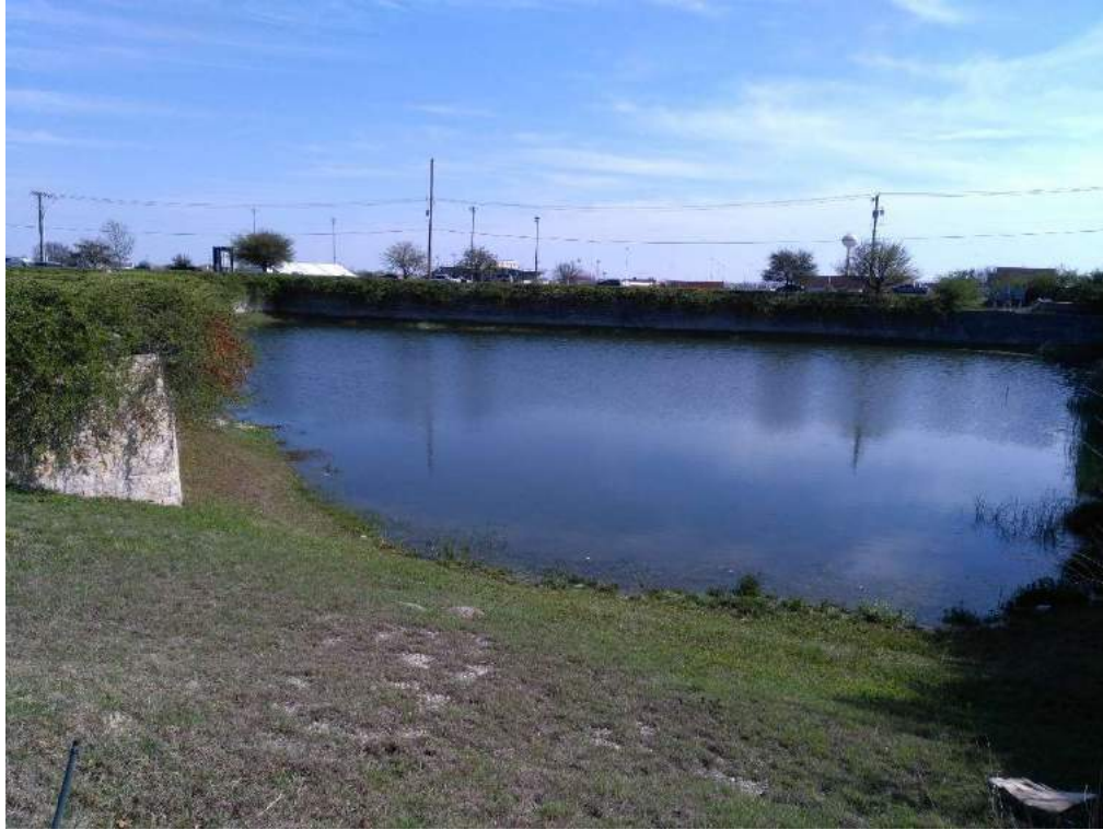
OVERALL VIEW OF DETENTION POND (LOOKING SOUTH)
