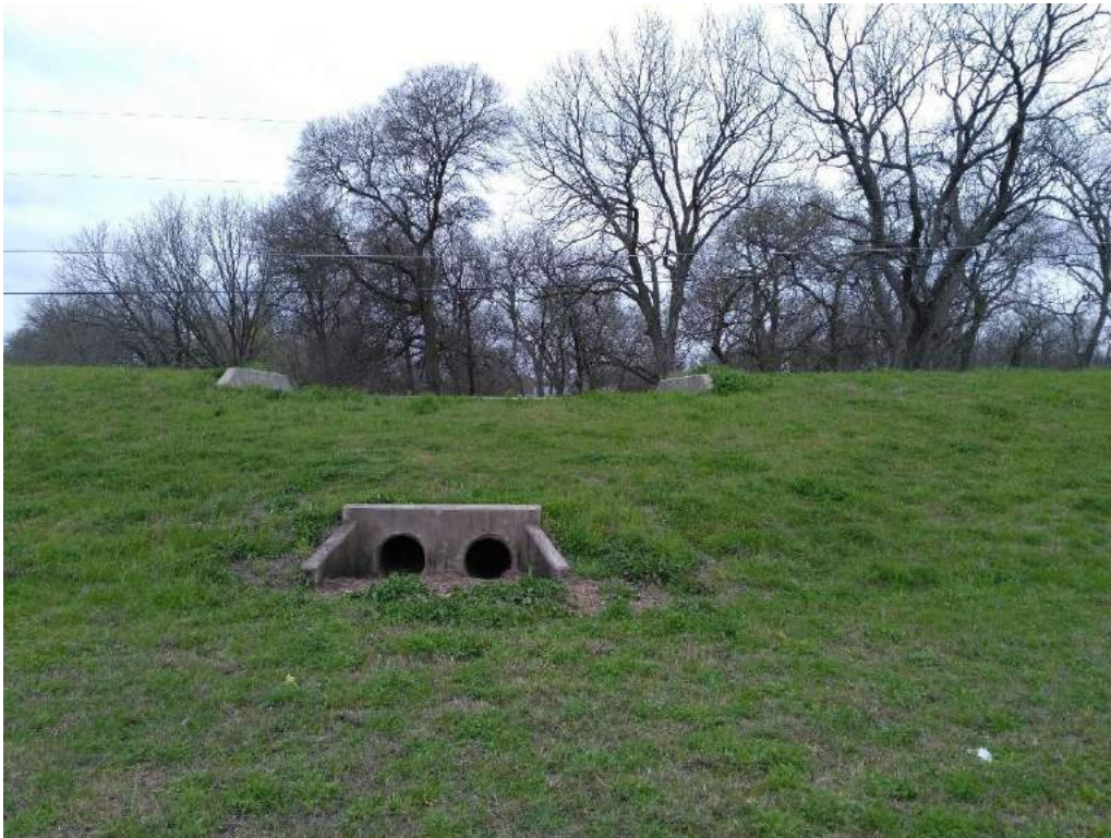
OVERFLOW STRUCTURES (LOOKING FROM UPSTREAM)
