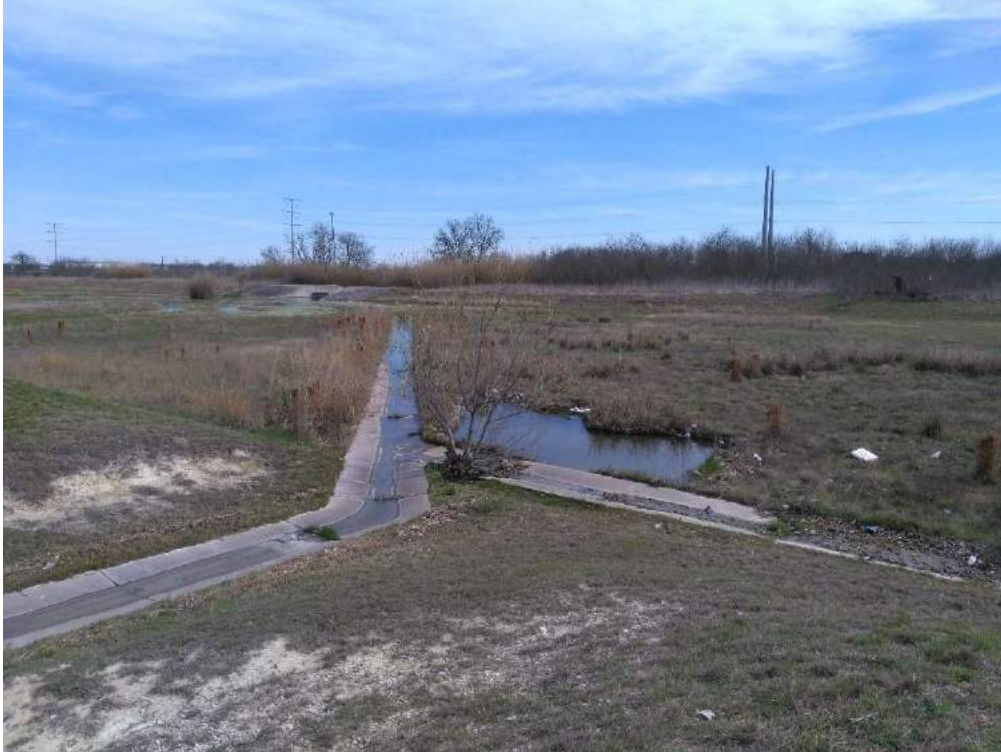
OVERALL VIEW OF DETENTION POND (LOOKING SOUTHEAST)
