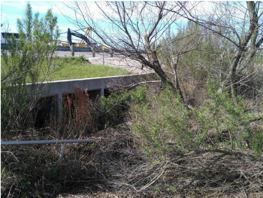
LOOKING DOWNSTREAM FROM OVERFLOW STRUCTURE
