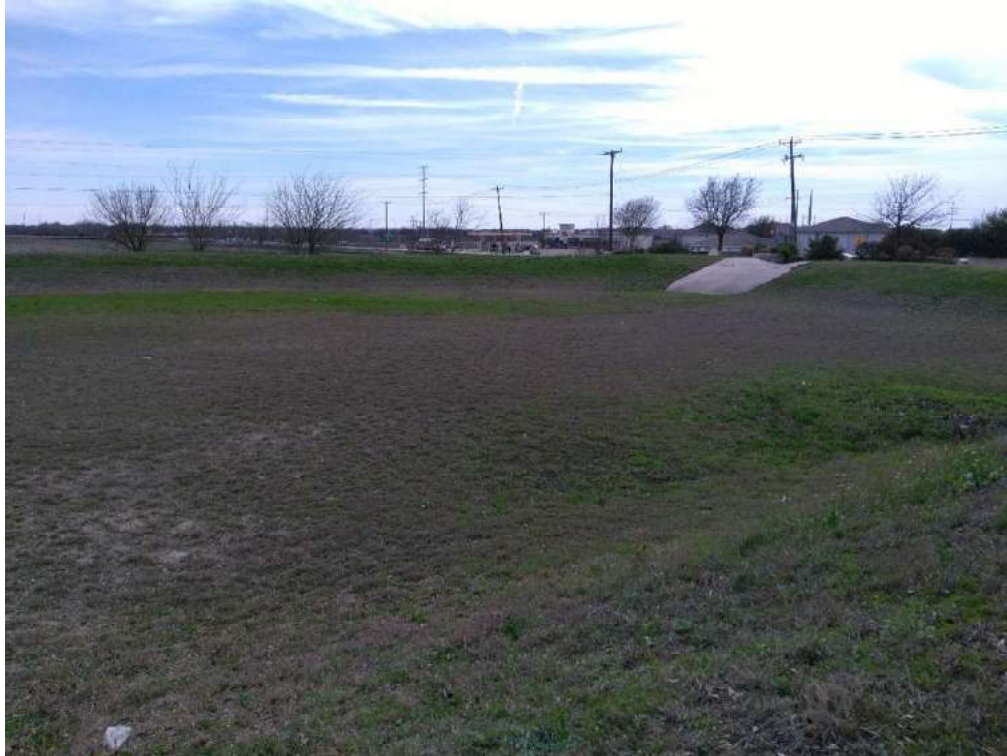
OVERALL VIEW OF DETENTION POND (LOOKING SOUTHWEST)
