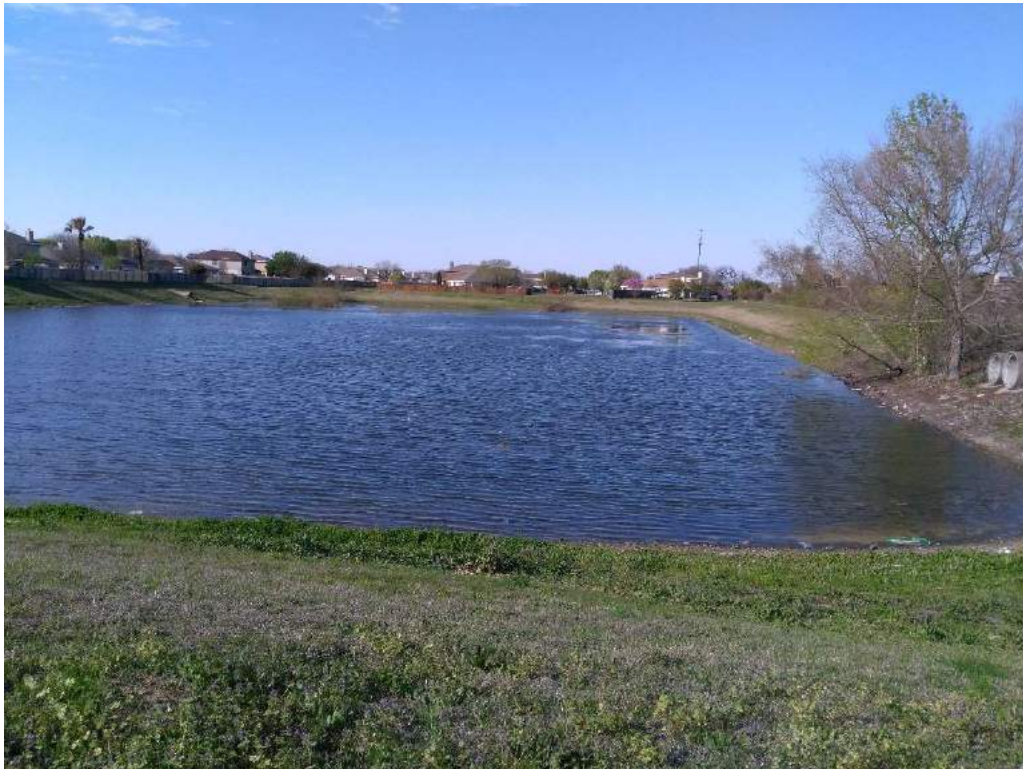
OVERALL VIEW OF DETENTION POND (LOOKING NORTH)
