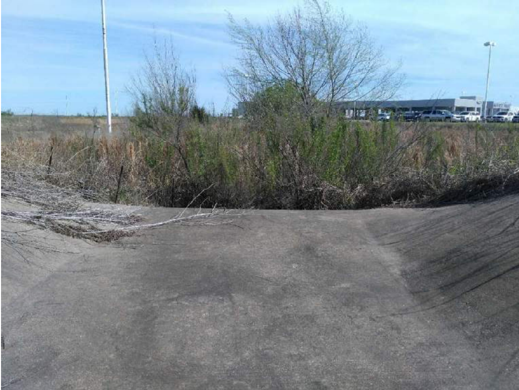
OVERALL VIEW OF DETENTION POND (LOOKING NORTH AT OVERFLOW STRUCTURE)
