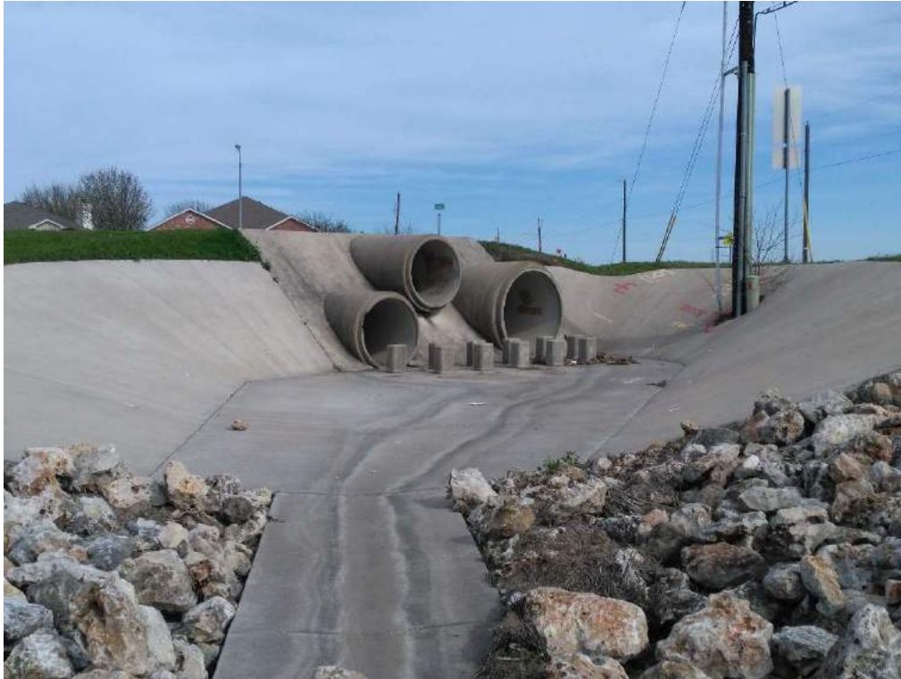
OVERFLOW STRUCTURE (DOWNSTREAM SIDE)
