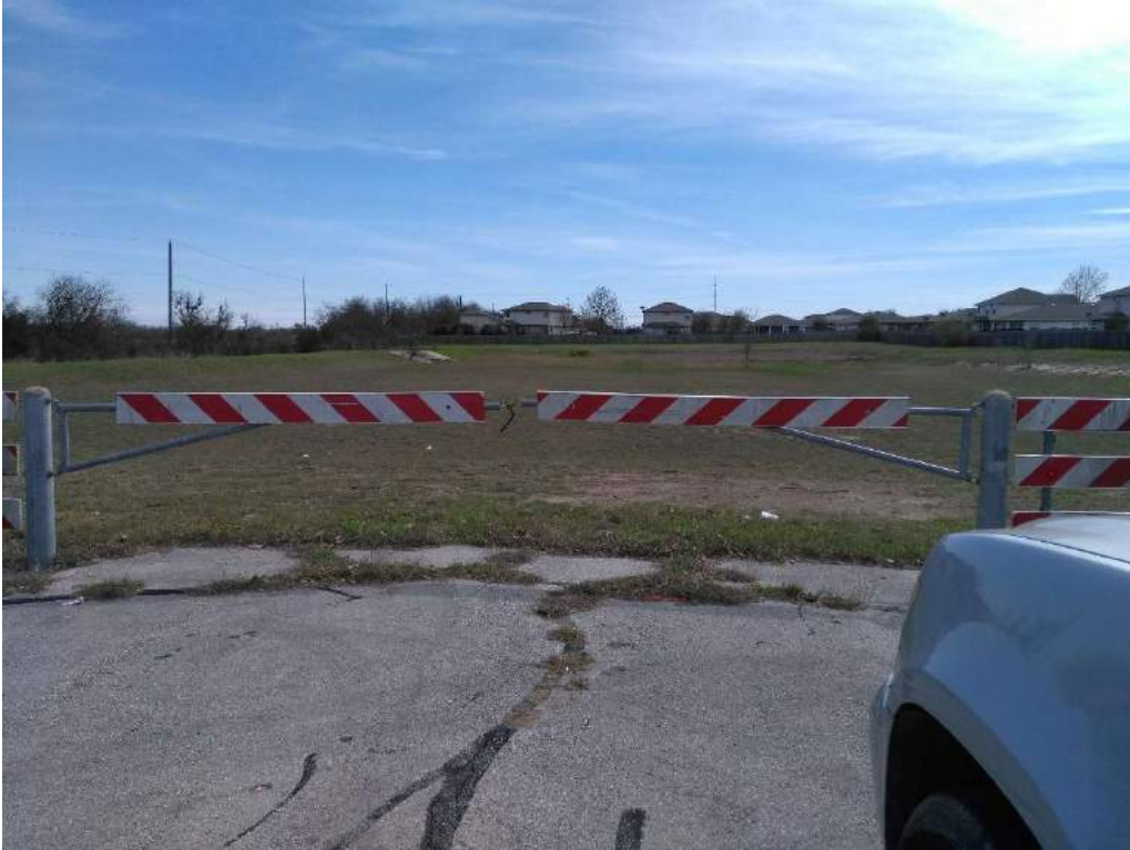
OVERALL VIEW OF DETENTION POND (LOOKING SOUTH)
