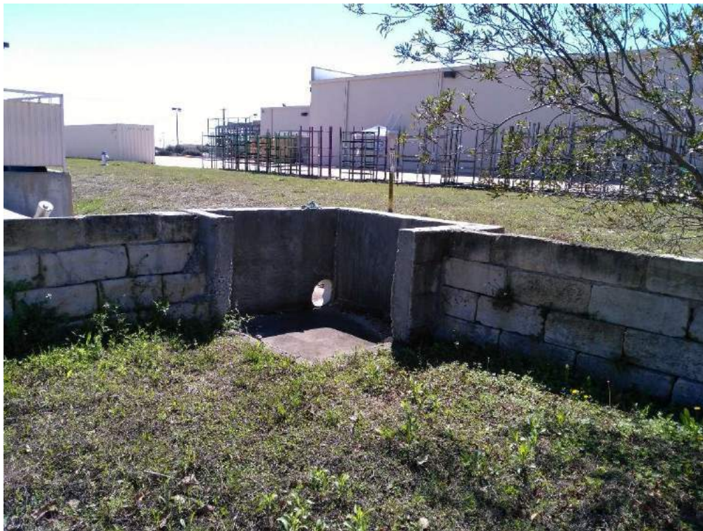
OVERFLOW STRUCTURE (LOOKING SOUTHEAST)
