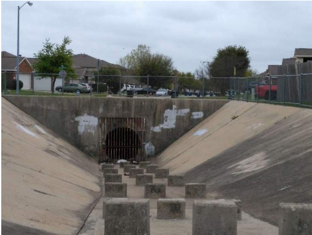
LOOKING DOWNSTREAM AT OVERFLOW STRUCTURE (NOTE SAFETY GRATE AT CULVERT)
