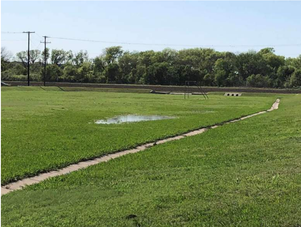
DETENTION POND (LOOKING SOUTH)
