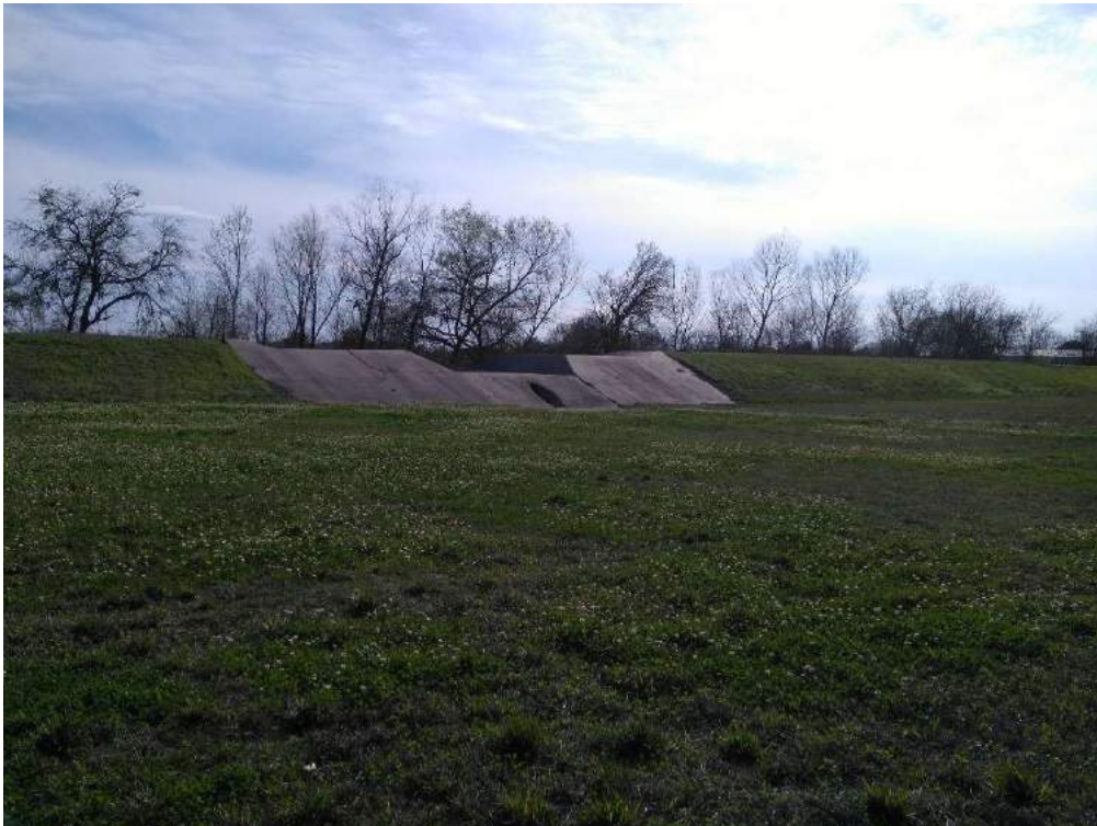
OVERALL VIEW OF DETENTION POND (LOOKING SOUTH)
