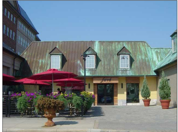
Outdoor patio, display windows
