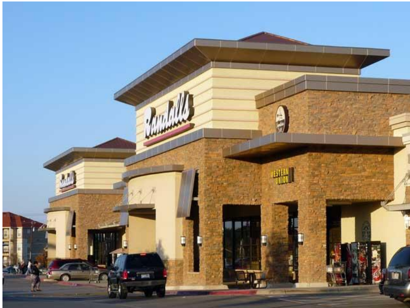
Well-defined building entrance
