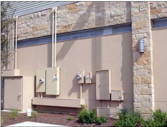
Utility equipment at back of building painted to match wall
