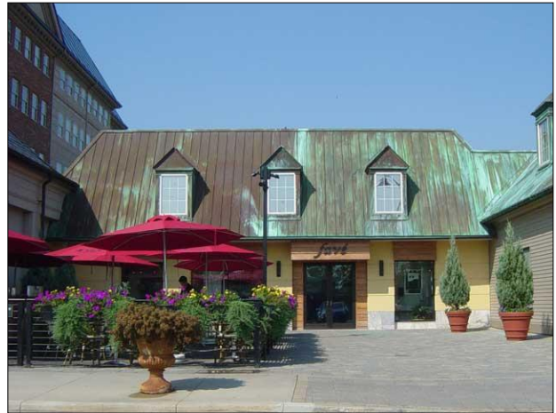
Outdoor patio, display windows
