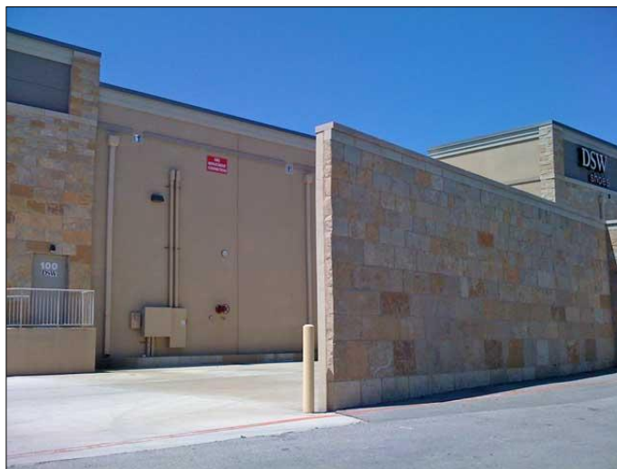
Effective use of wing wall used to screen loading dock
