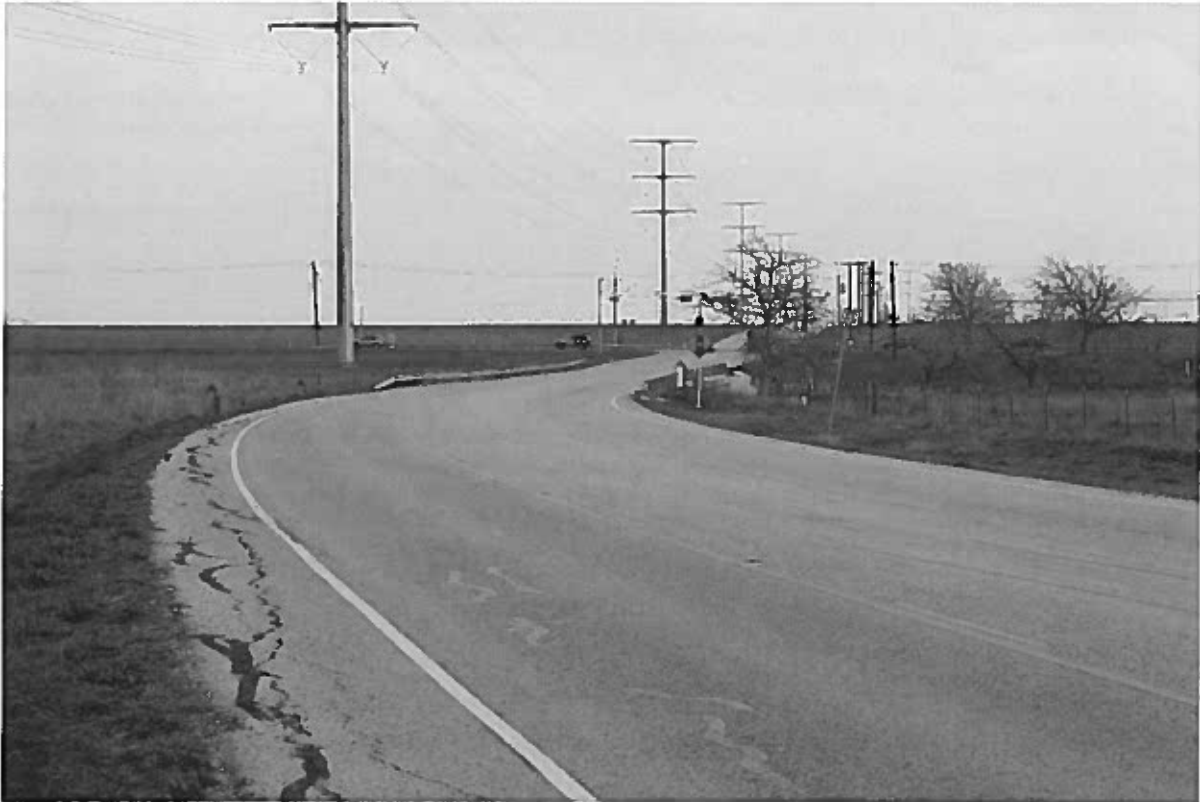
Photo 1 – Looking east towards the Limmer Loop and FM 1660 Intersection (Please note the Box Culverts at Limmer Loop crossing over Cottonwood Creek)
