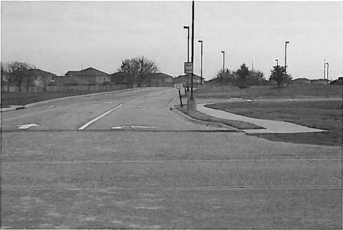
Photo 4 – Looking south on the northside of Limmer Loop at the Cottonwood Creek Elementary and Hutto Middle School driveway where proposed sidewalk would tie into school sidewalk
