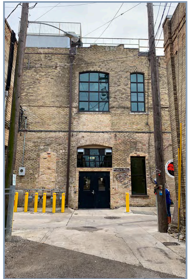
Alley-entrance to an art studio in Taylor, TX, provides interest, expands the use of the building, and activates an alley.
