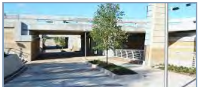
Tunnel connecting Texas A&M campus under an active railroad and street. Klotz Associates.
