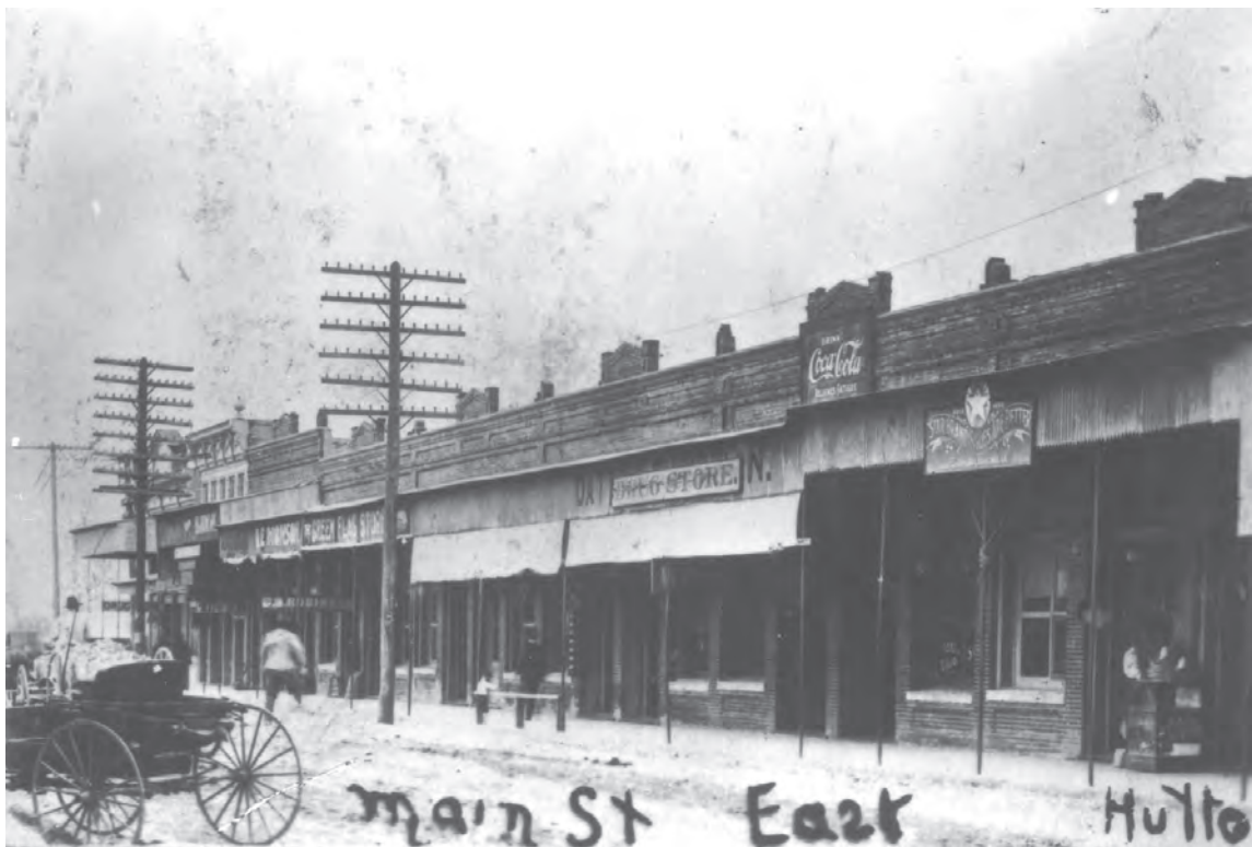
Photograph of buggy and people on Main Street in downtown Hutto. Main Street 1890 building on corner of Highway 79 and East St. General merchandise and bank building. 5
