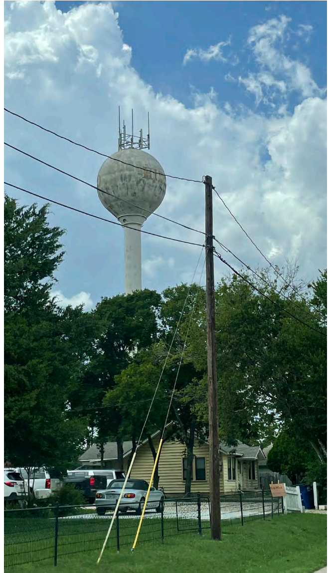
Water Tower & Electrical Lines
