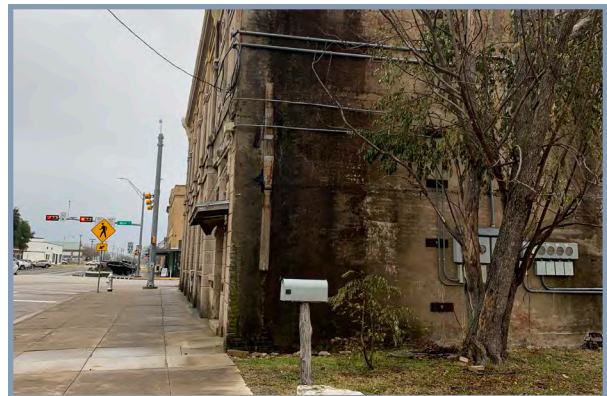
Regular maintenance to remove bio growth on areas prone to moisture is necessary for masonry.
