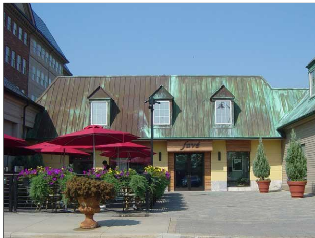
Outdoor patio, display windows
