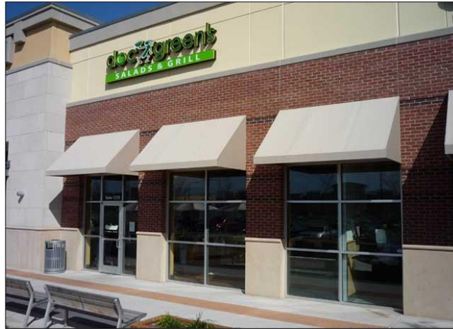
Separate awnings above individual windows
