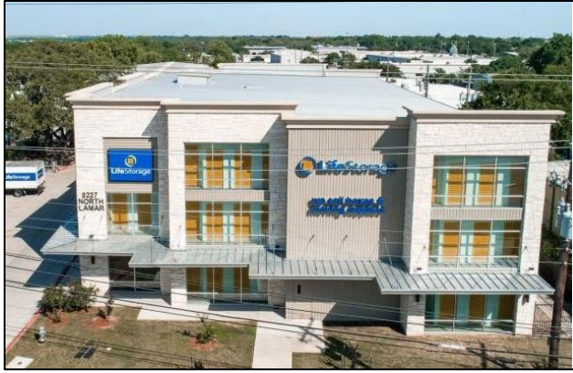
Building with flat roof incorporating a parapet. First story articulated with metal eave overhang. Façade articulation.
