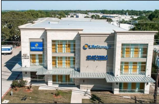
Building with flat roof incorporating a parapet. First story articulated with metal eave overhang. Façade articulation.
