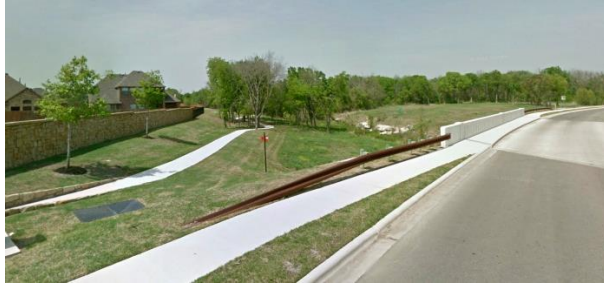
Wide concrete trail graded for bike and pedestrian use within linear open space area accessible from street, undisturbed wooded and natural area and perimeter stone wall
