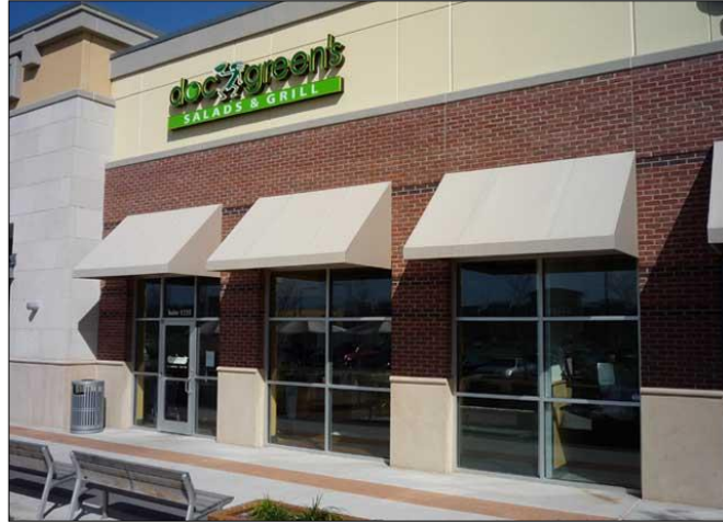
Separate awnings above individual windows
