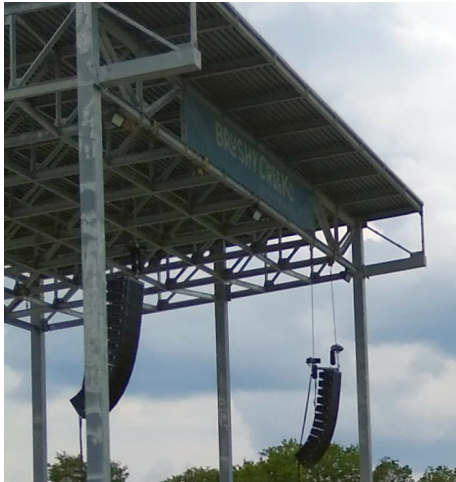
Figure 5.1 Needed speaker hang height and venue roof height. Hanging subwoofers may not be an option unless the hang goes lower.
