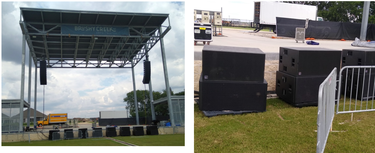
Figure 4.2: Sound System for Field Test. Left, subwoofer array along the front of stage and line arrays suspended. Right, subwoofers stacked: lower system is the cardioid directional subwoofers and upper system is the traditional more omnidirectional subwoofers.
