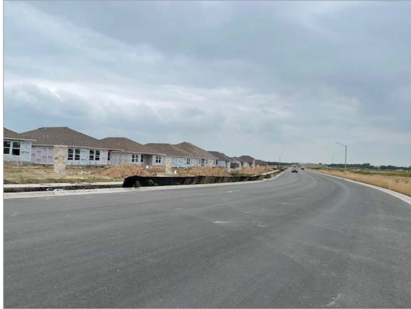
Homes Under Construction in Platted Cottonwood Phase 1
