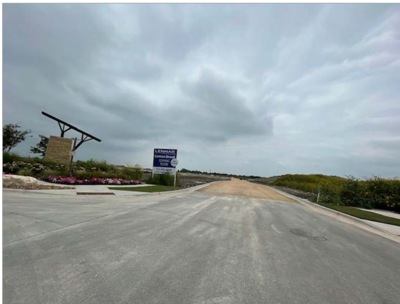
Extension on Carl Stern Drive Under Construction
