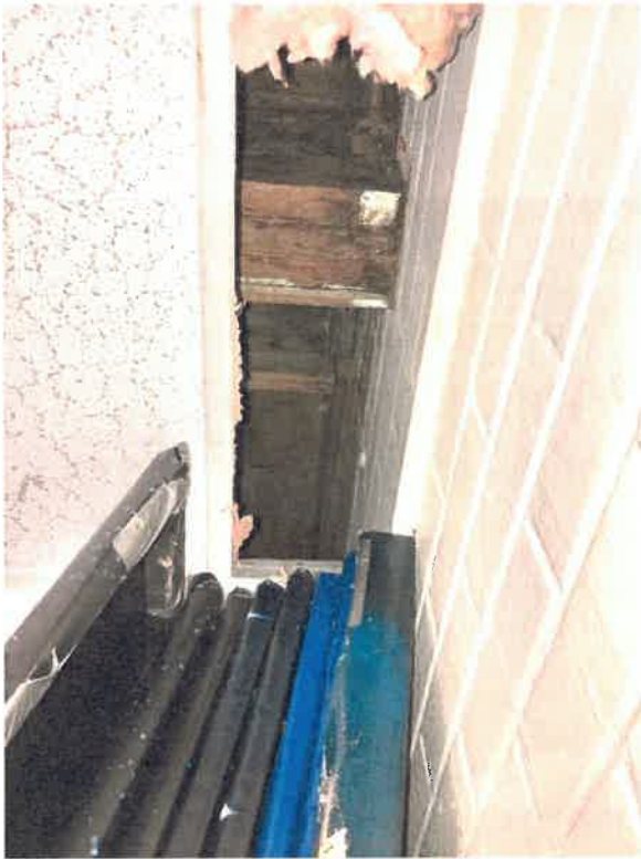
Photo 2 - North side building, looking up at wood beam.
