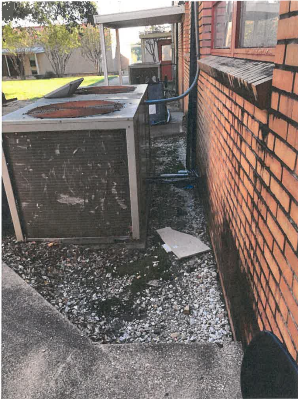
Photo 20 - North wall of the Gym as seen from the exterior, looking East.
