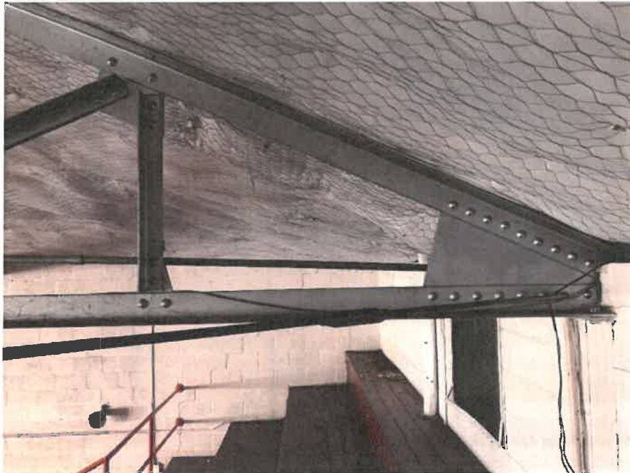
Photo 9 - End of the Westernmost Gym roof truss at the North wall.
