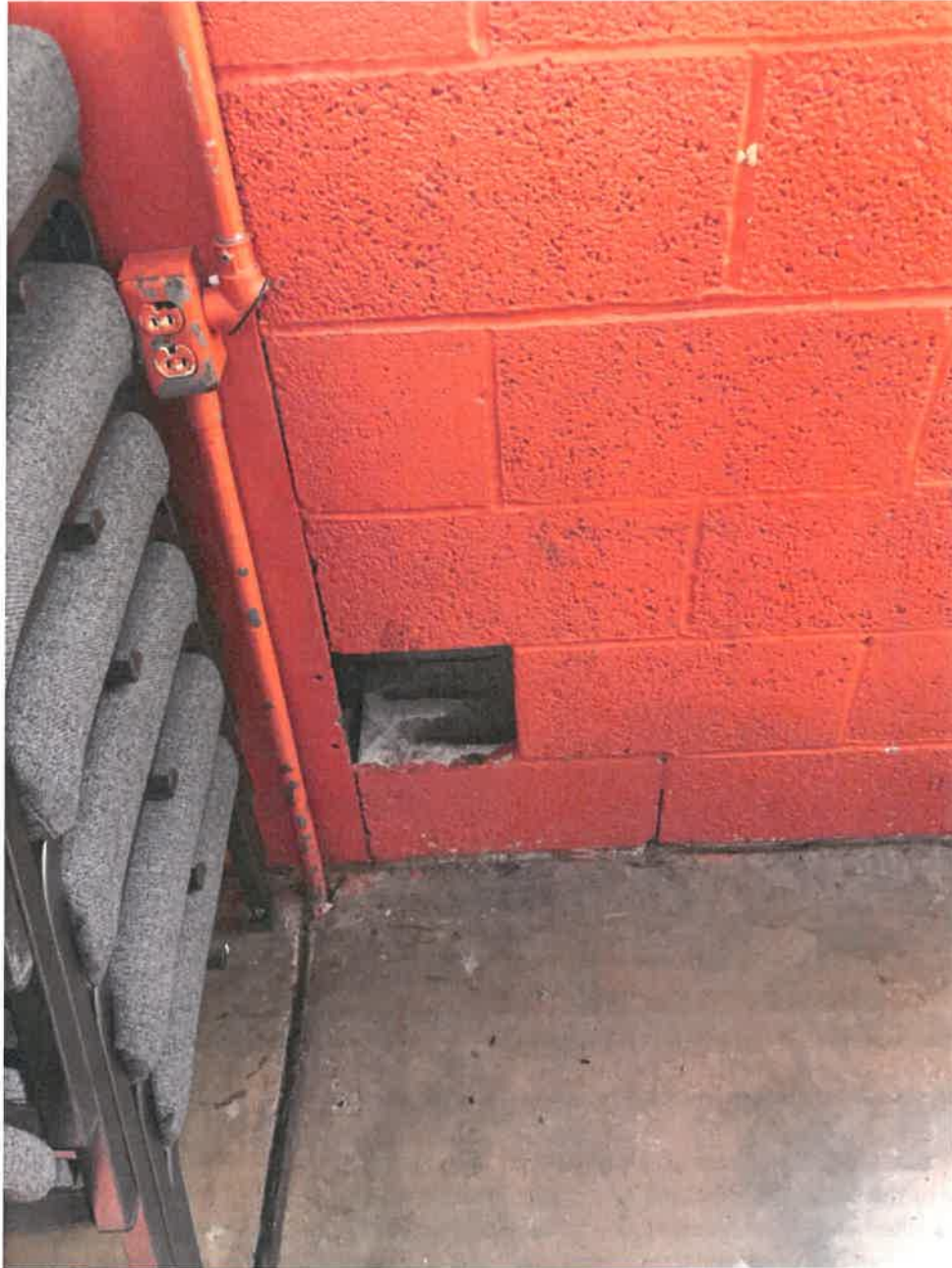
Photo 13 - Base of column near along the South wall of the Gym.
