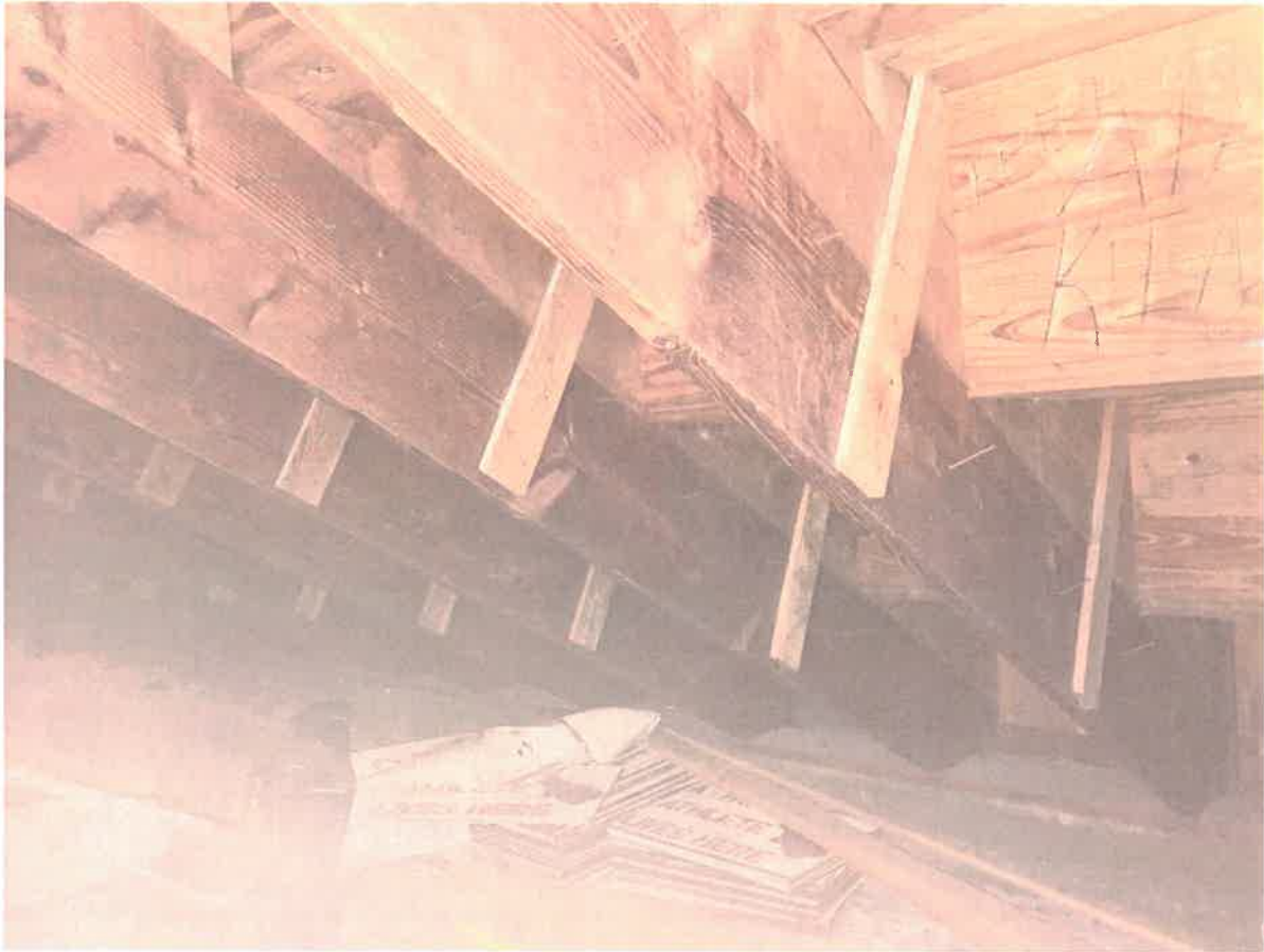
Photo 23 - Underside of bleachers near access door, looking South.
