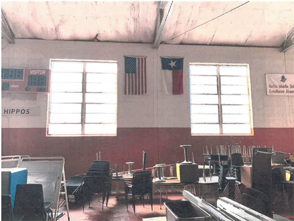
Photo 14 - South wall of the Gym as seen from center-court, looking South.
