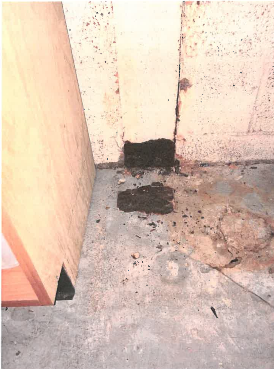
Photo 18 – Easternmost column base at North wall near.
