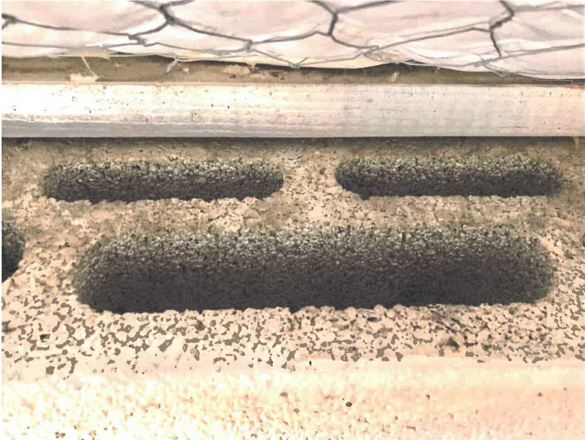
Photo 12 - Top of CMU wall at the North side of the Gym as seen from top of bleachers.
