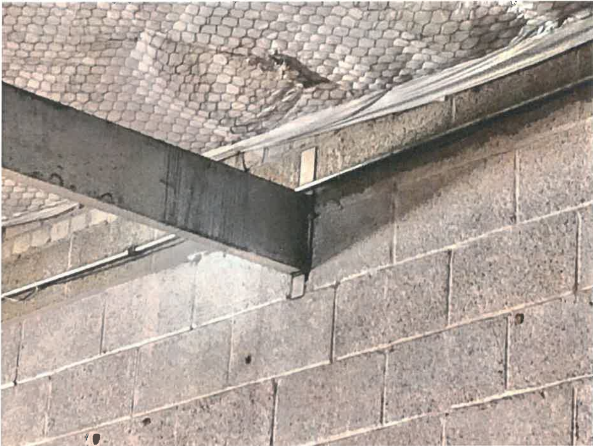
Photo 11 - West wall of Gym looking from top of bleachers.
