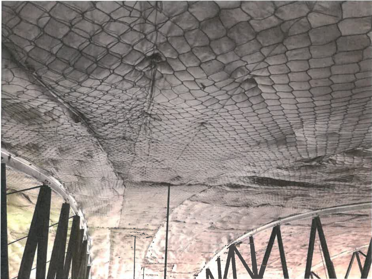
Photo 6 - Underside of Gym roof as seen from the North wall, looking South.
