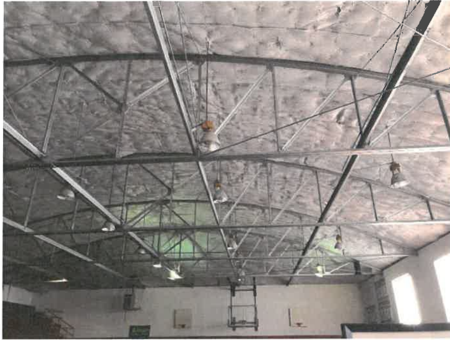
Photo 8 - Underside of Gym roof structure, looking East.
