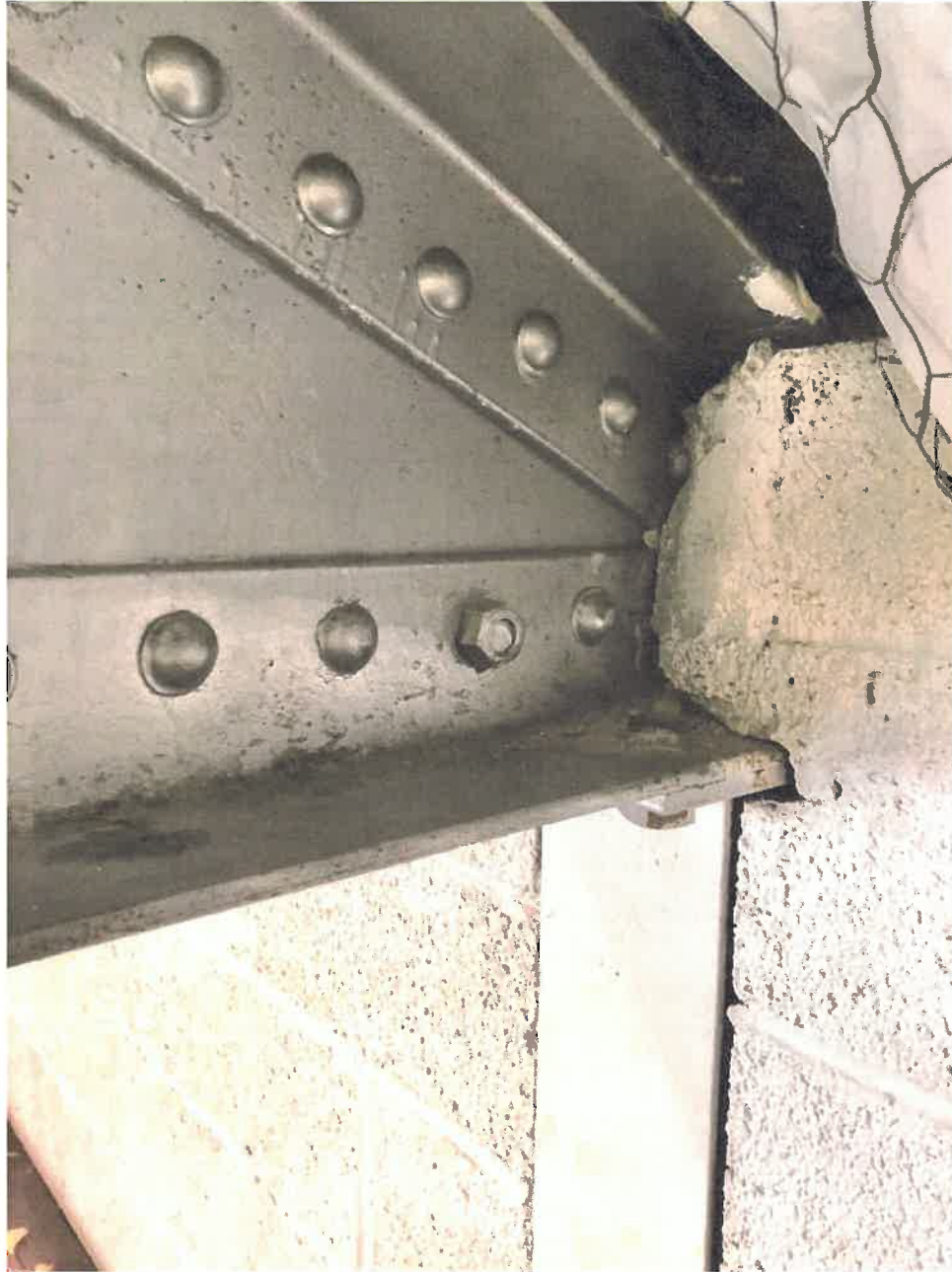
Photo 10 - Gym roof truss connection to column at the North wall.
