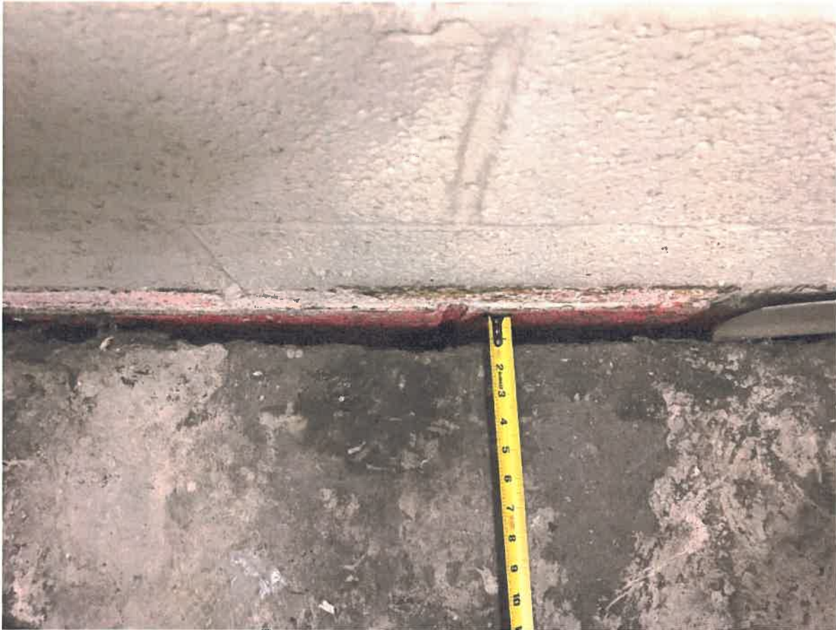
Photo 19 - Base of North wall near _____.
