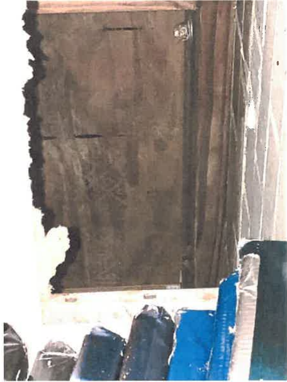
Photo 3 - North side building, looking up at wood ledger and wood decking.
