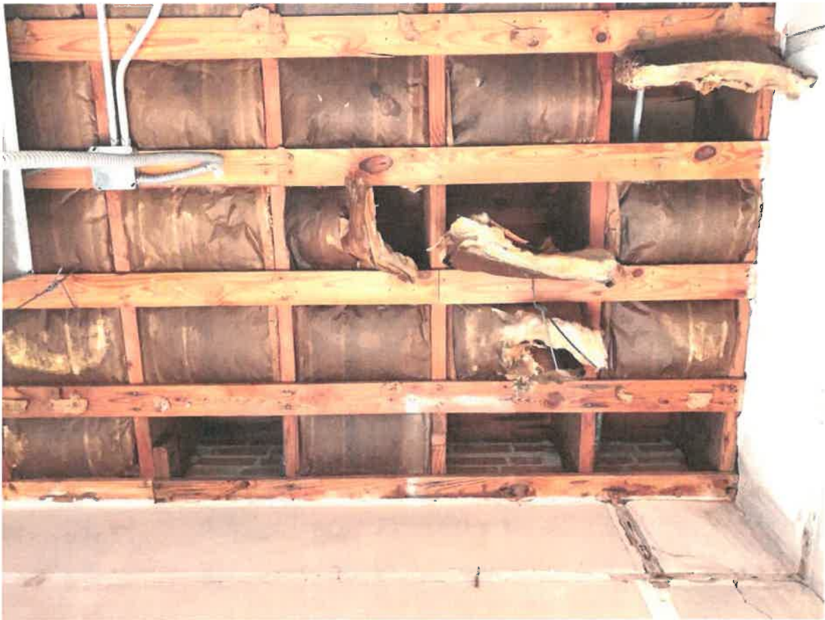
Photo 4 - West side locker room building, looking up at wood roof rafters and brick facade.
