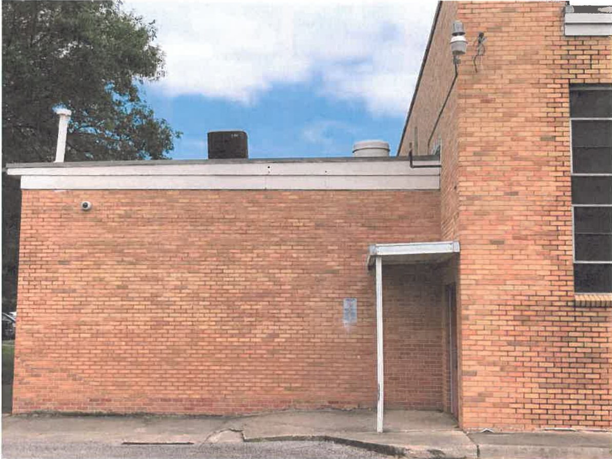
Photo 5 - Exterior of the West side locker room building as seen from the South.
