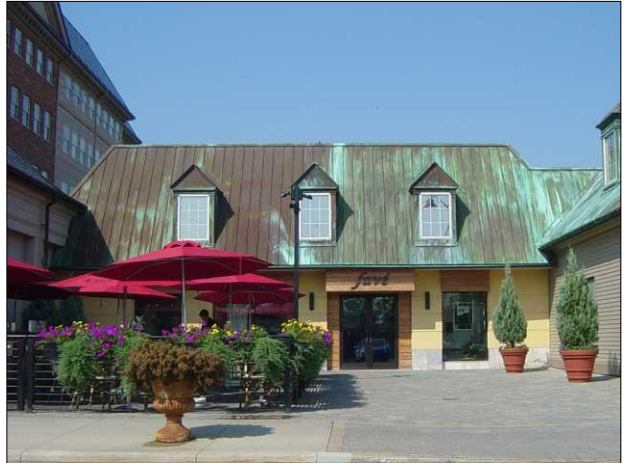
Outdoor patio, display windows
