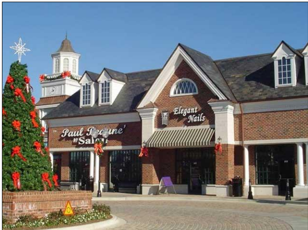
Peaked roof form, canopy, display windows, projections
