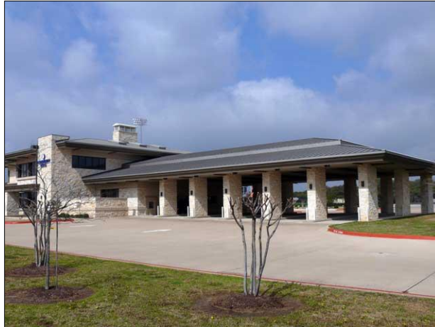
Drive-through architecturally integrated into host structure
