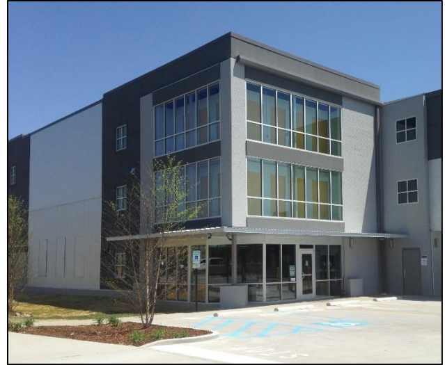
First floor articulation at office entry. Contemporary material use of articulated glass and metal and rhythm of building massing.
