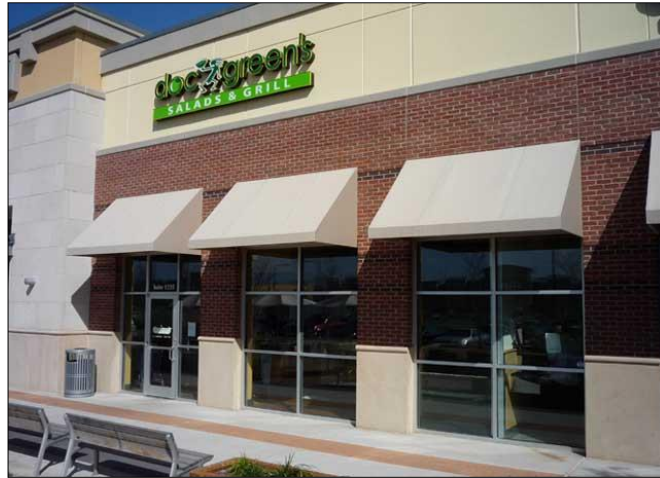
Separate awnings above individual windows
