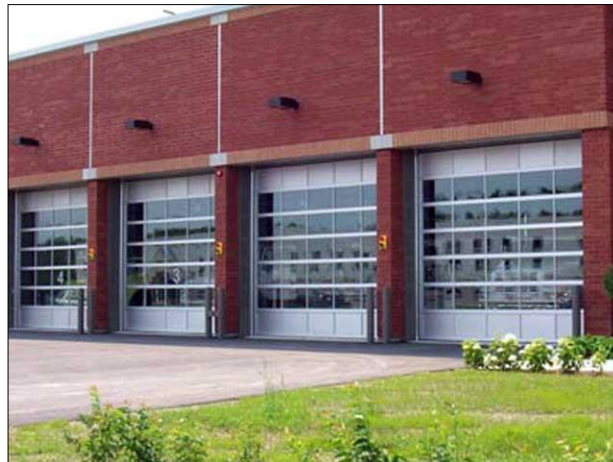
Garage doors integrated into building architecture
