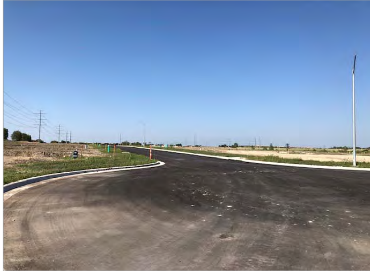
Infrastructure in Place
