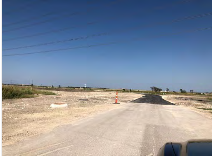
Secondary Entrance Off Ed Schmidt Boulevard
