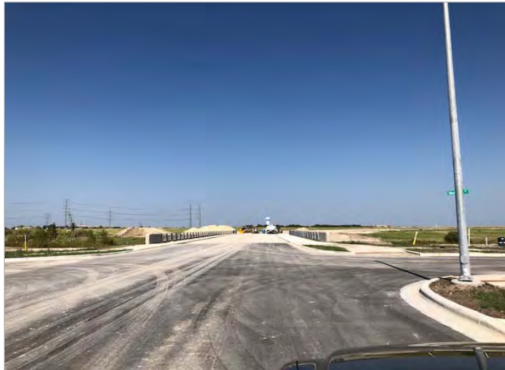
Infrastructure with Bridge Over Floodplain
