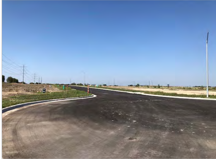
Infrastructure in Place
